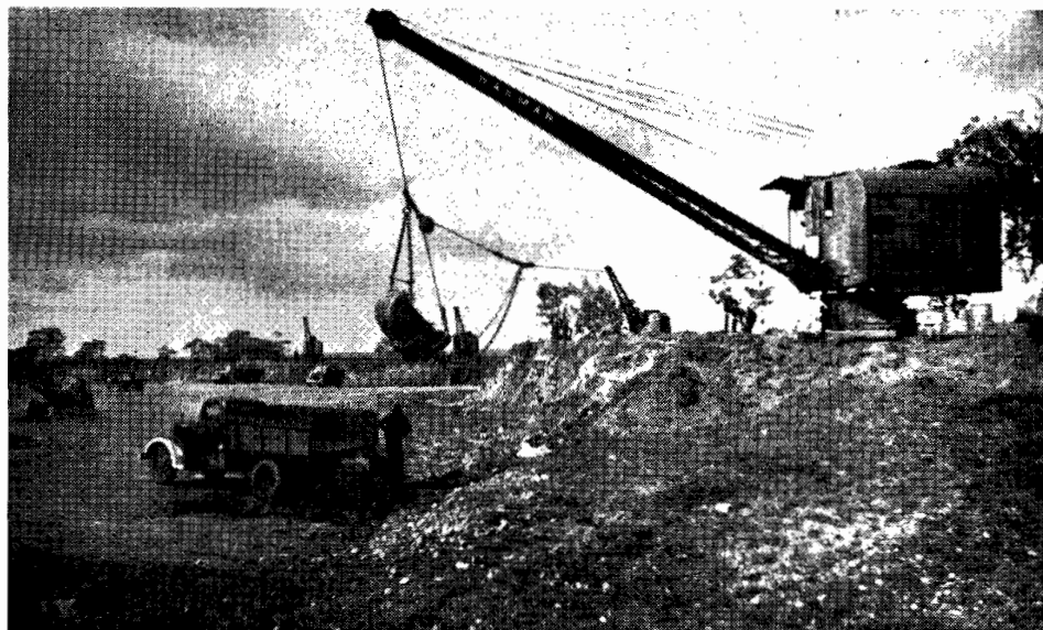
PLATE 25.—Winning gravel for construction of runways at East Sale.
