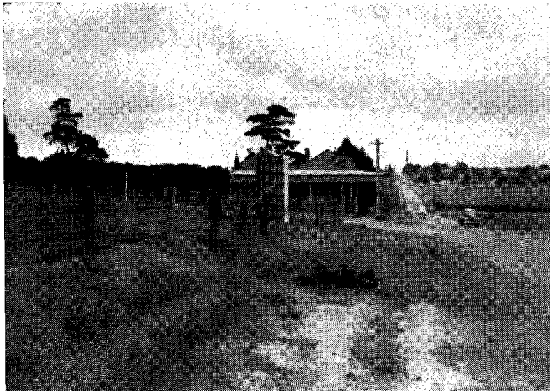
PLATE 10.—Warrigal Road-Waverley Road intersection, showing building acquired as part of widening scheme.
