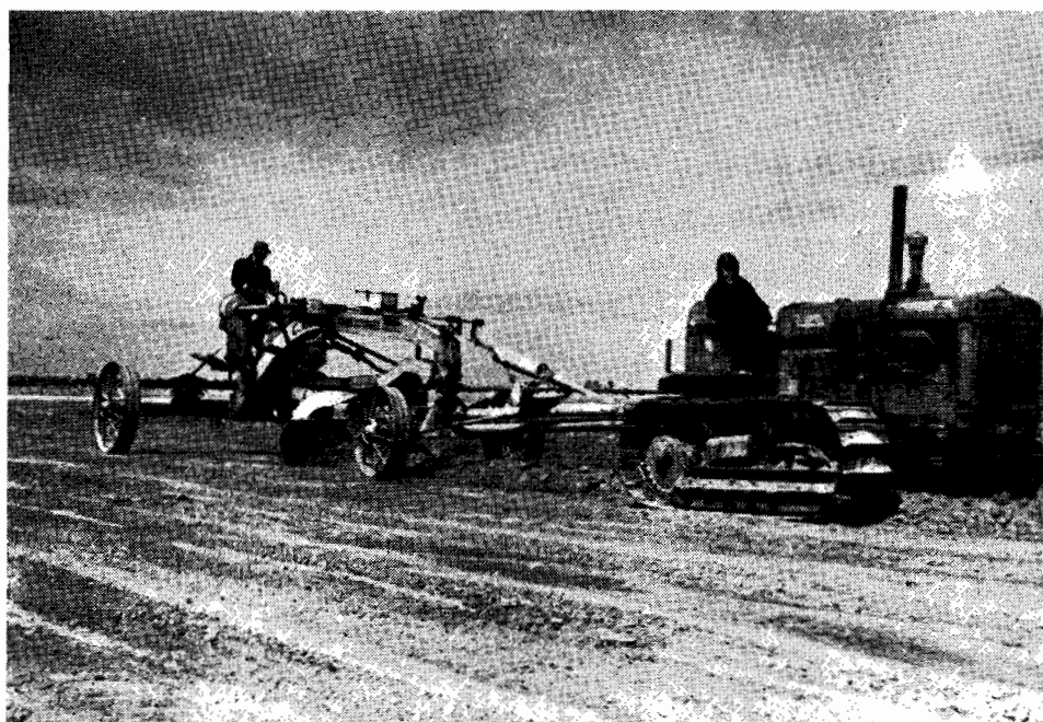
PLATE 26.—Spreading gravel on runways, East Sale.
