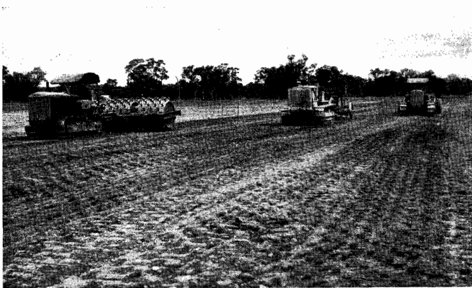
PLATE 24.—Construction of runways, Mangalore West.
