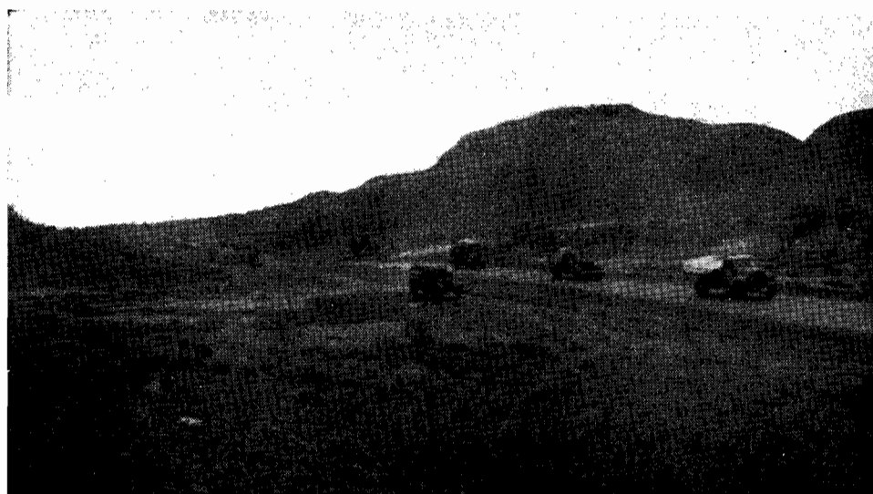
PLATE 18.—Completed section of Stuart Highway near Tennant Creek, showing military convoy.
