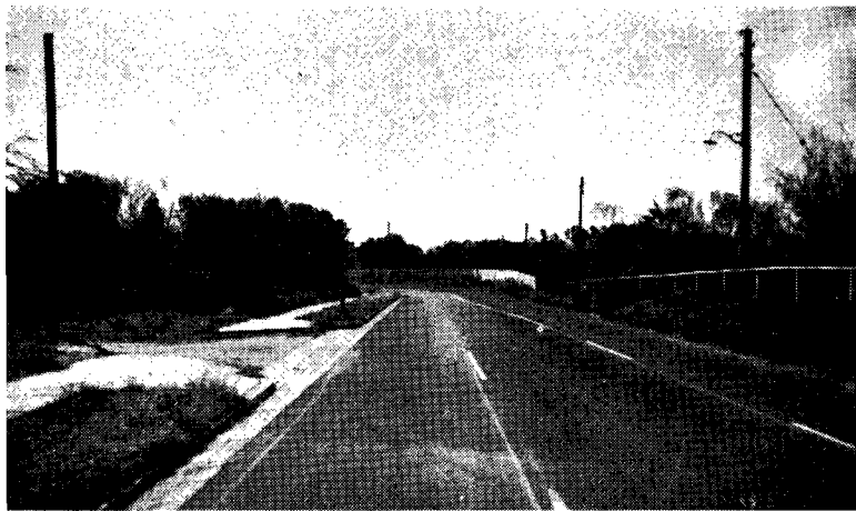
PLATE 11.—Sandringham City, Beach Road, showing restricted visibility at "Jackson's Corner" before clearing.
