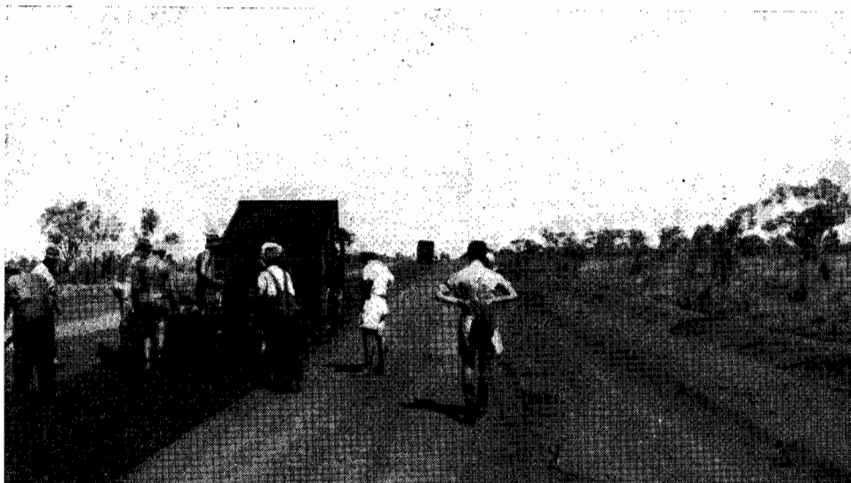
PLATE 16.—Spreading bituminous macadam wearing course on Stuart Highway near Tennant Creek.
