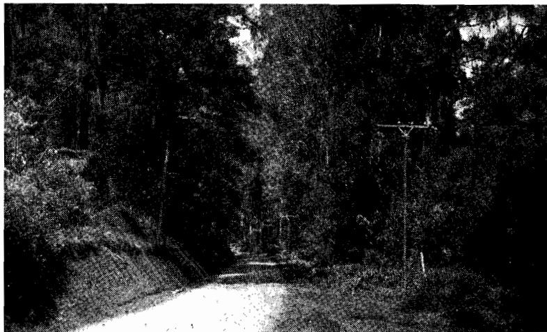
PLATE 5.—Healesville Shire—Myers Creek Road showing section of reconditioned road.
