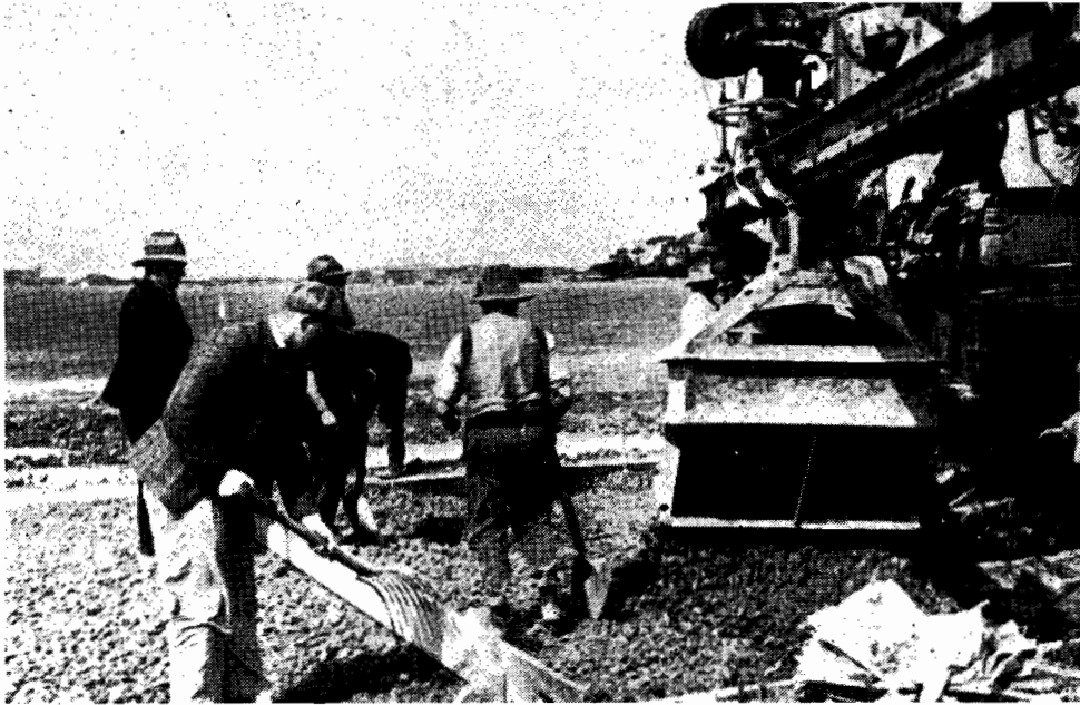
PLATE 23.—Construction of concrete runways, Point Cook aerodrome.
