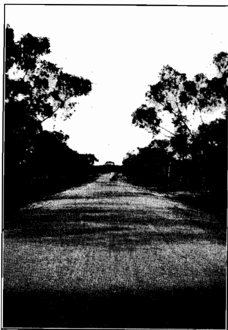
Plates Nos. 3 and 4.—Showing Henty Highway between Hopetoun and Lascelles before and after reconstruction.
