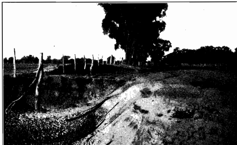
Plate No. 15.—Showing scour at flood crossing caused by floods in the Shire of Charlton.
