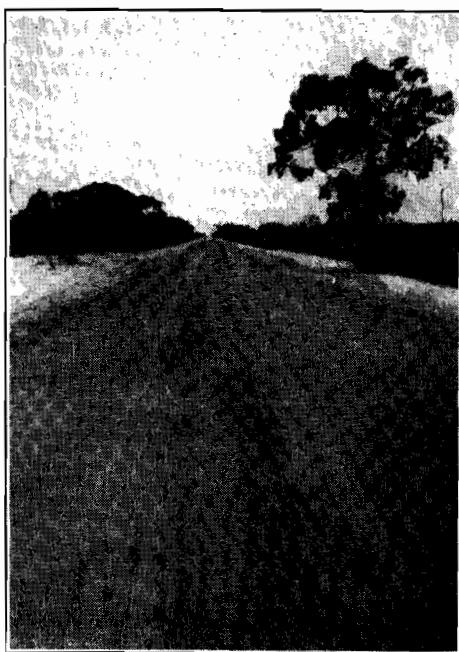
Plate No. 5.—Kaniva-Edenhope-road after treatment with common salt.
