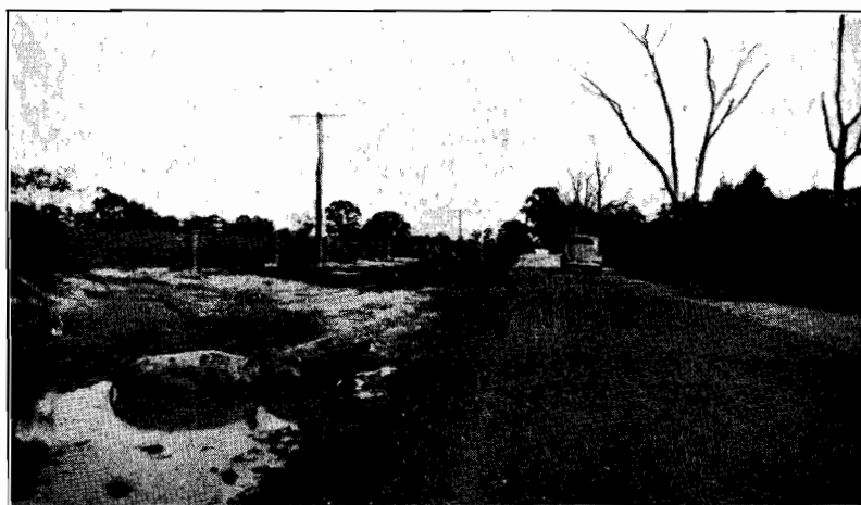
Plates Nos. 6 and 7.—Showing result of excavating on the roadsides for borrowing soil for road formation.
