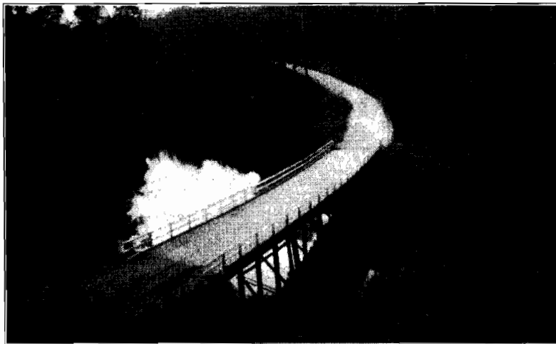
Plate No. 25.—Showing new bridge erected on the Princes Highway East over the Toorloo Arm.
