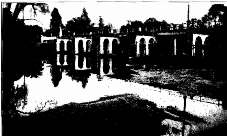
Plate No. 26.—Showing work in progress for the widening of the bridge over the Broken River on the Sydney Road at Benalla.
