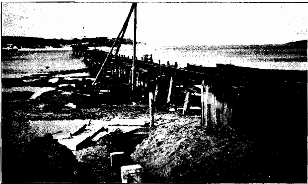
Plate No. 28.—Showing progress of work on the above bridge at the 30th June, 1939.
