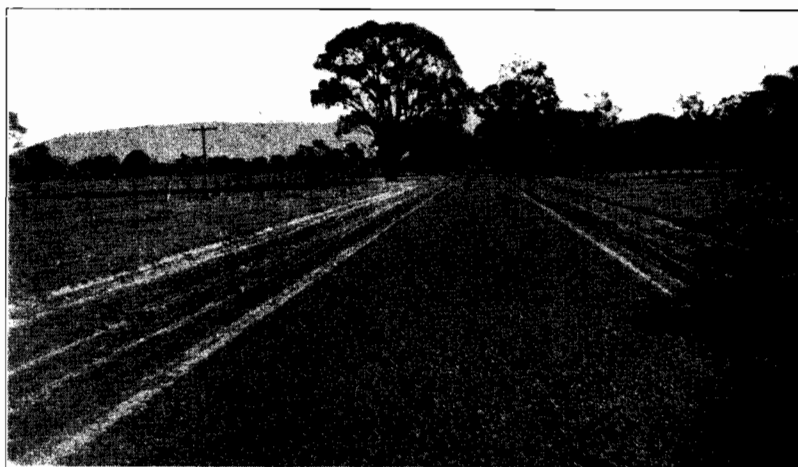
Plate No. 20.—Showing Grampians Road gravelled and sealed between Mt. Emu and Hall's Gap.
