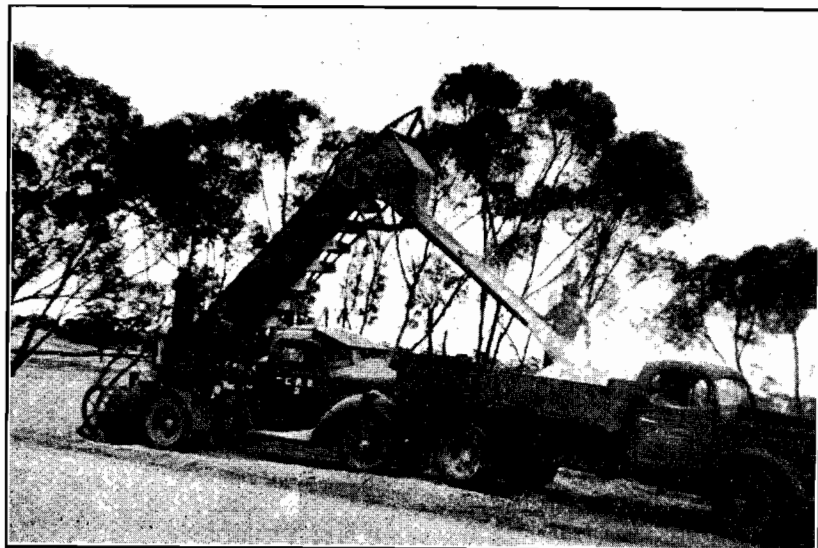
Plate 41.—Showing Aggregate Loader in Operating Position.
