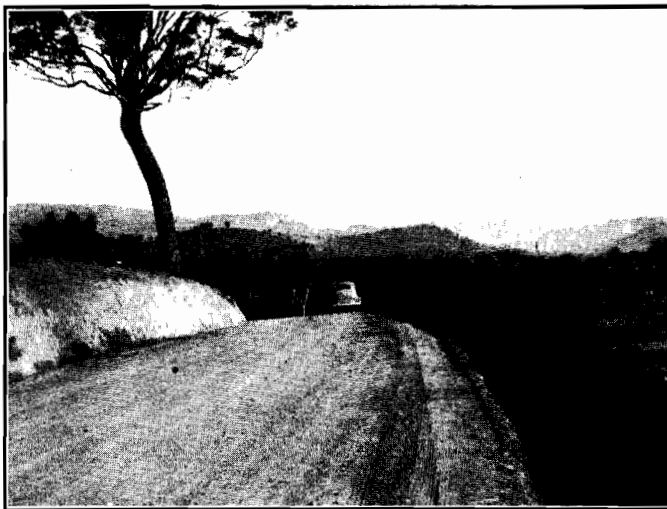
Plate No. 3.—Showing improved alignment between Granya and Thologolong on the Murray Valley Highway.
