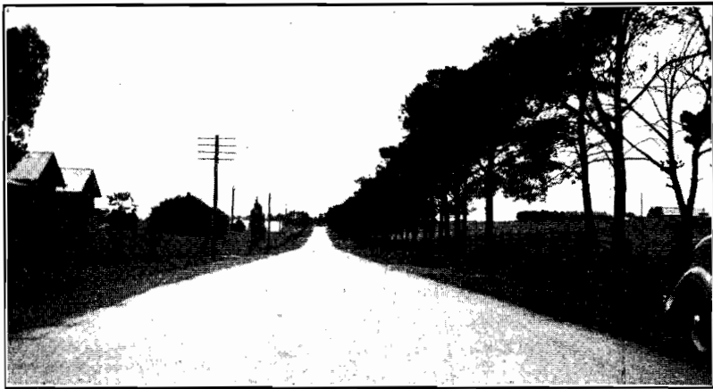
Plate No. 18.—Showing type of work completed on Cordite Avenue leading to the Munition Factory at Maribyrnong.
