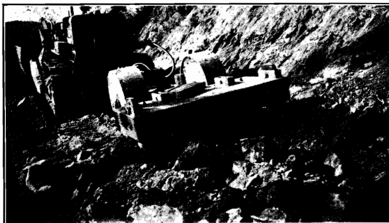
Plate No. 50.—Ripper with tynes lowered being drawn by a crawler tractor.
