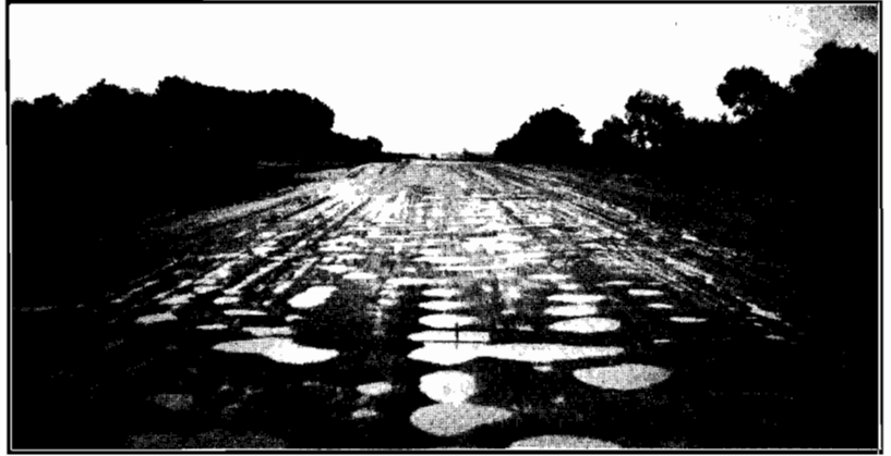
Plate No. 7 is an example of neglected maintenance of a constructed road.
