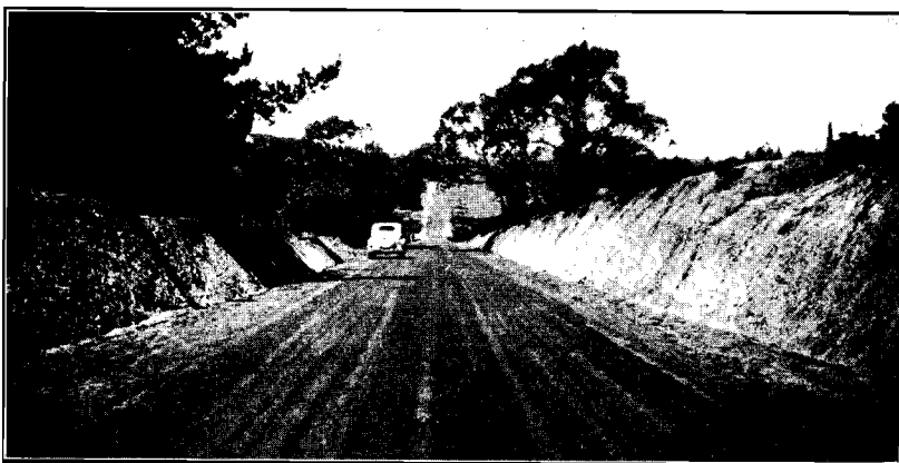
Plate No. 15.—Showing completed work on the Newington-Ocean Grove Road.
