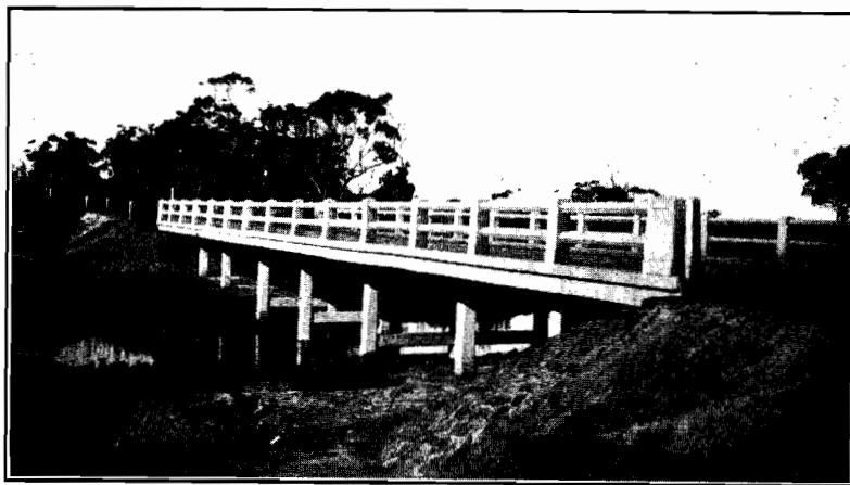
Plate No. 23.—New bridge erected over Darlot Creek on the Prince's Highway West.
