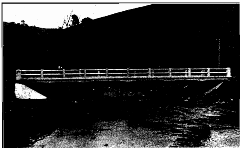
Plate No. 27.—Showing new bridge erected over Little River at Taggerty.
