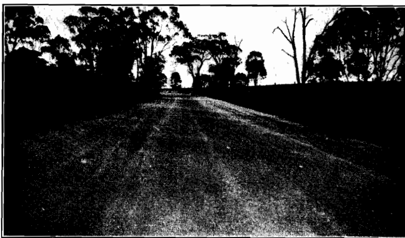
Plate No. 9.—Showing reconstructed section of the Goulburn Valley Road in the Shire of Goulburn.
