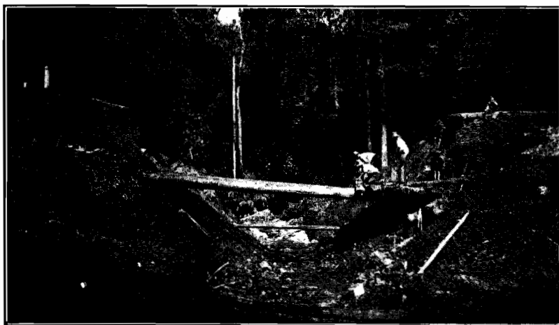
Plate No. 1.—Washout at Euchre Creek Valley.
