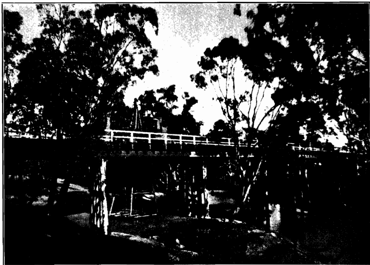
Plate No. 25.—Bridge over the Loddon River at Serpentine.
