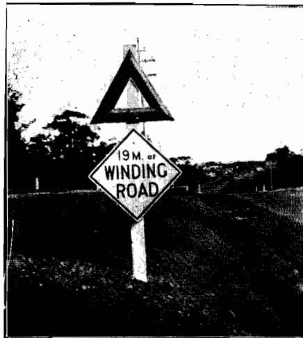
Plate No. 42.—Showing new type of warning sign.
