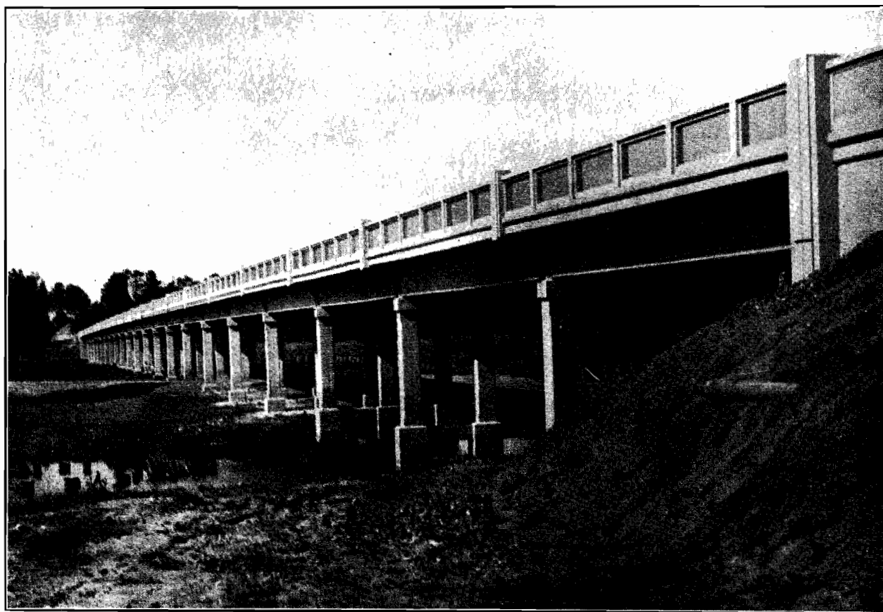
Plate No. 22.—New bridge erected over the Latrobe River and adjacent flats at Rosedale.
