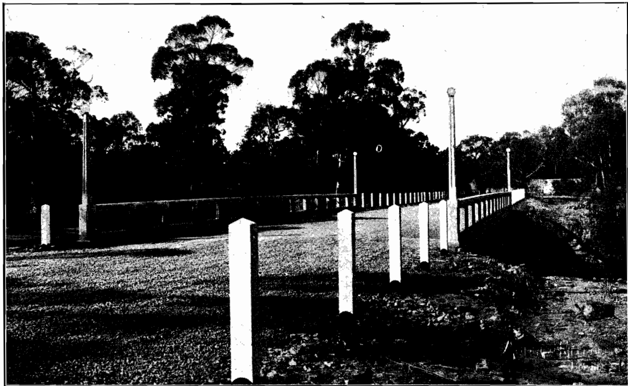
Plate No. 28.—New bridge erected over the Dandenong Creek on the Burwood Road.
