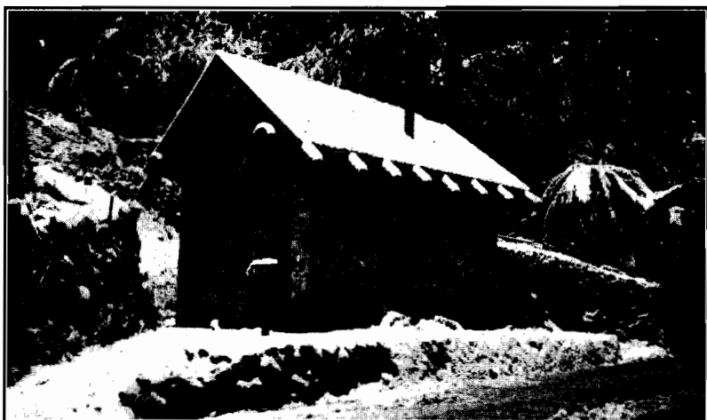
Plate No. 32.—Showing sanitary accommodation provided on the Acheron Way. Photograph was taken after a fall of snow.
