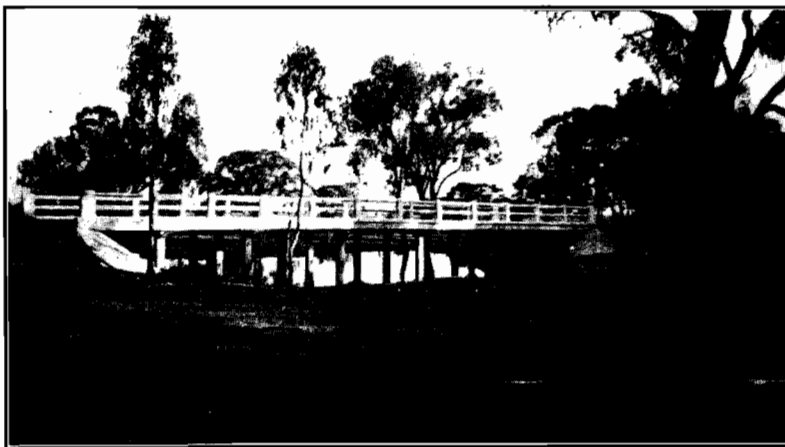
Plate No. 26.—Showing new bridge erected on the Echuca-Cohuna Road in the Borough of Echuca.
