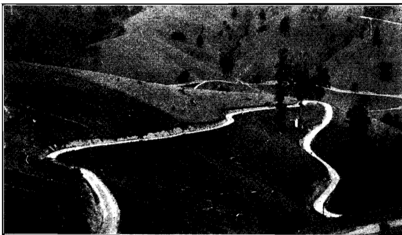
Plate No. 17.—Isolated settler's road known as Henry's Road in the Shire of Alberton.
