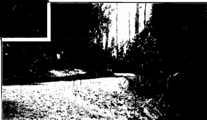
Plate No. 18—Illustrating type of country through which the Noojee-Erica Road is being constructed, and Plate No. 19—Completed section of forming under a light covering of snow on the same road.
