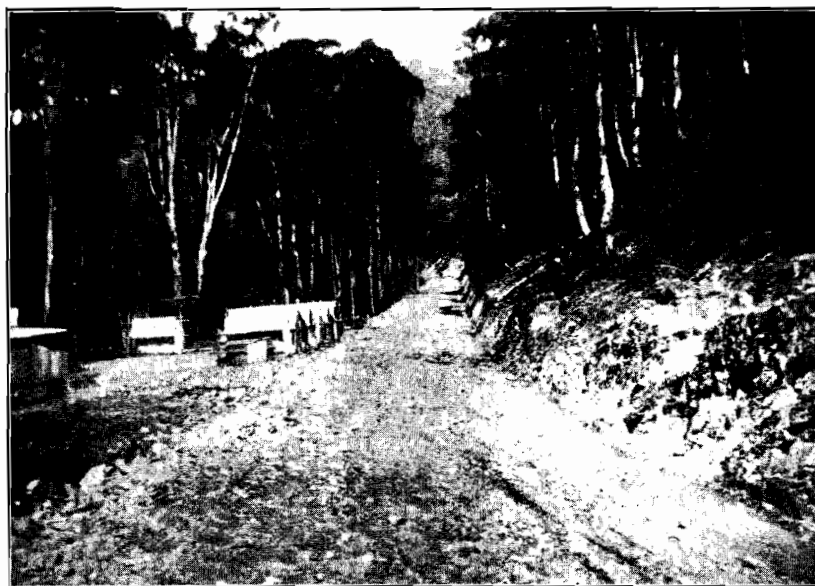
Plate No. 15.—Partially constructed section of Eildon Weir-Jamieson Road, between Peachey's Bridge and Woods Point Road.
