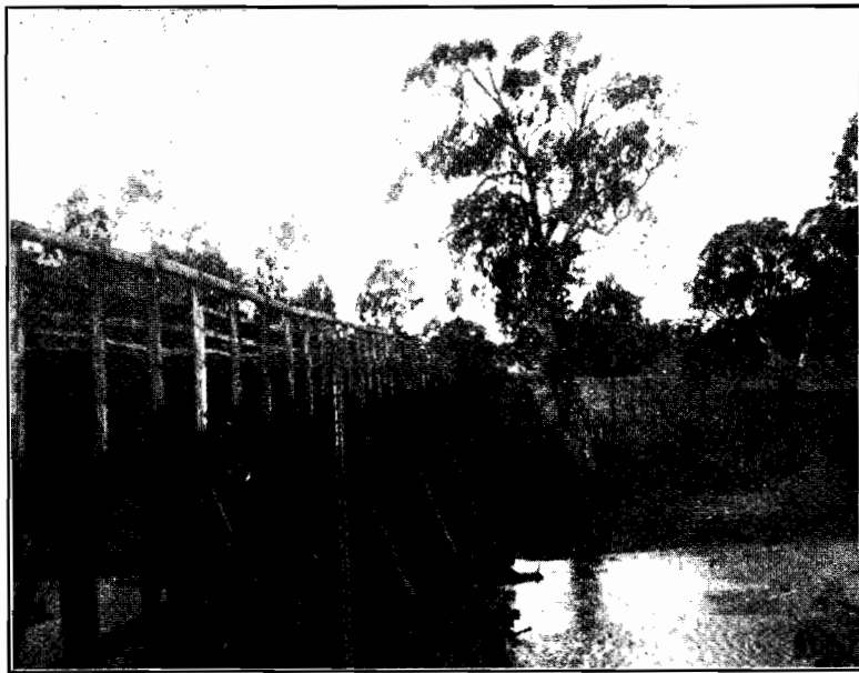
Plate No. 24.—Showing the Old Bridge over the Loddon River at Newbridge.
