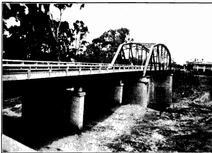
Plate No. 23.—New bridge over the Goulburn River at Murchison.
