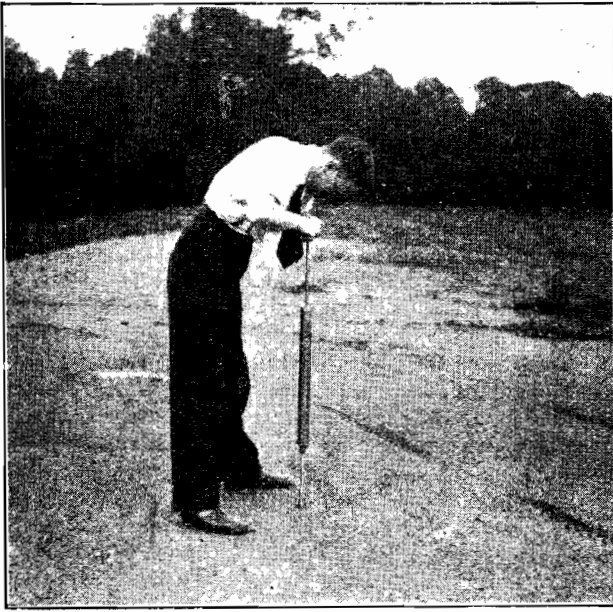
Plate No. 50.—Use of Proctor Penetration Needle in the Field.
