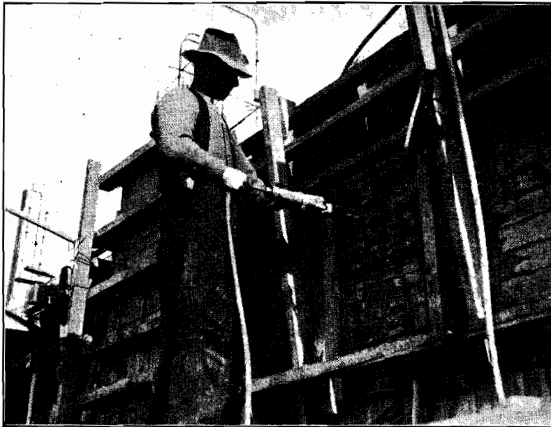
Plate No. 54.—Concrete Vibrator in Operation.
