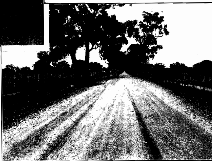
Plates Nos. 13 and 14.—Showing section of the Yarraberb Road before and after construction.
