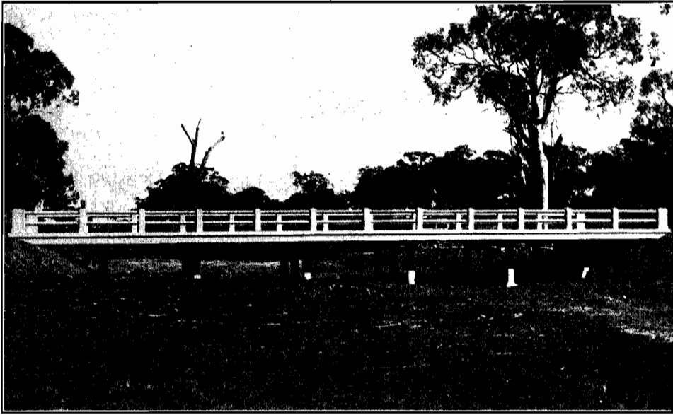
Plate No. 26.—New bridge over Stockyard Creek on the Benalla-Yarrawonga Road.
