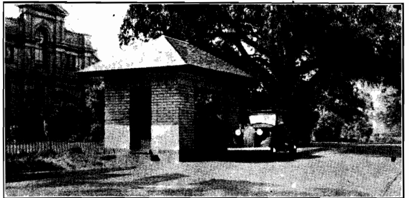
Plate No. 39.—Showing new weighbridge and office erected near Motor Registration Branch.
