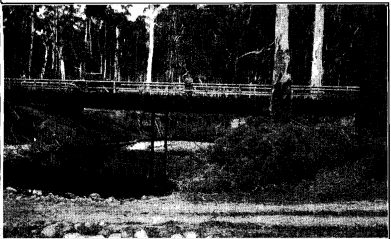
Plate No. 35.—Showing the New Bridge over Fyann's Creek, on the same road.
