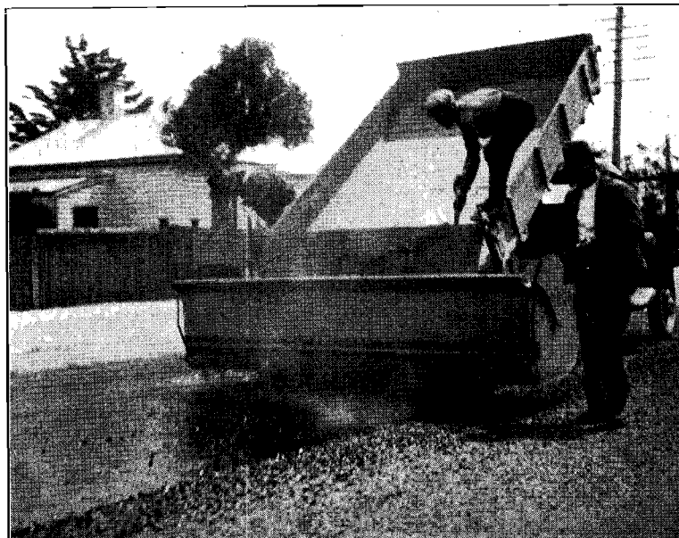
Plate 38.—“ Buckeye ” Spreader in Operation.
