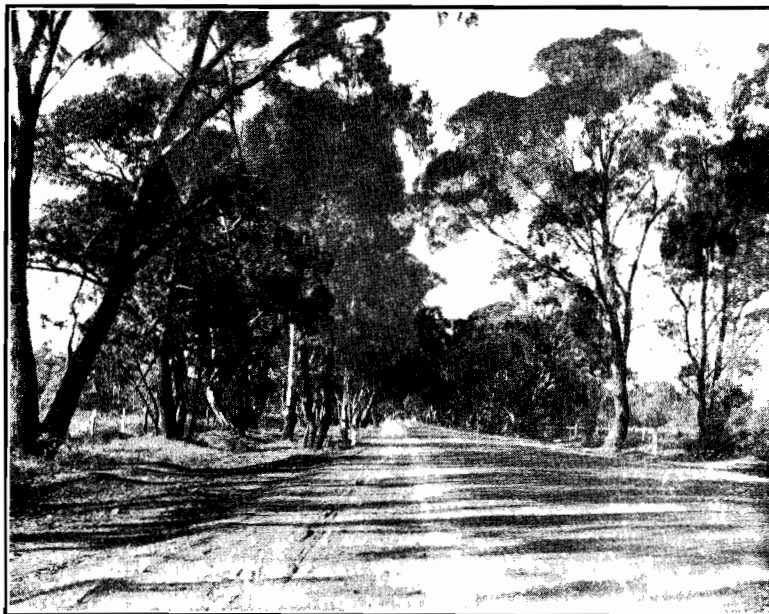
Plate No. 1.—Widened section of Calder Highway between Castlemaine and Bendigo.
