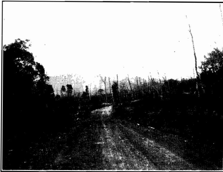
Plate No 17.—Showing work done on Rose River Road, Oxley Shire.
