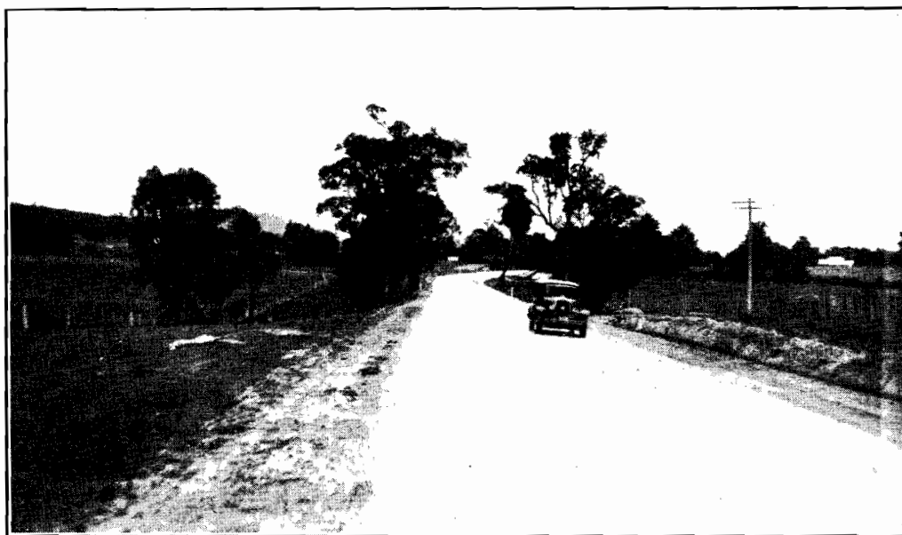
Plate No. 4.—Recent work done on the Midland Highway between Buninyong and Ballarat.
