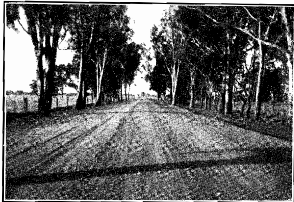
Plate No. 3.—Murray Valley Highway—Resheeting east of Rutherglen.
