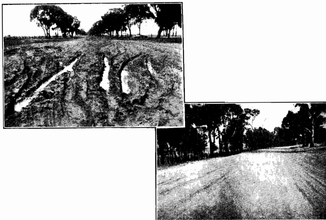
Plates Nos. 14 and 15.—Showing Benalla-Tocumwal Road before and after construction.
