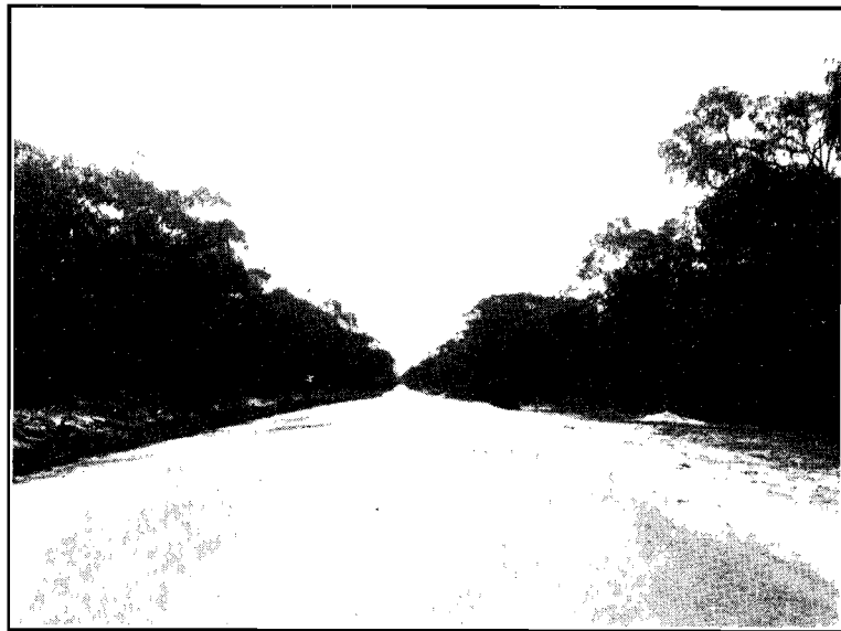
Plate No. 6.—Western Highway near Ararat, resurfaced with road-mix seal.
