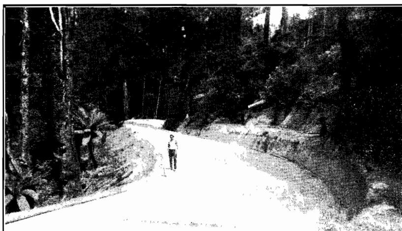
Plate No. 12.—Recently constructed Black's Spur deviation on the Healesville–Alexandra Road.
