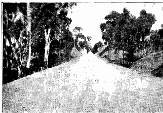
Plate No. 22.—Widened section of Midland Highway, near Maindample Turnoff.
