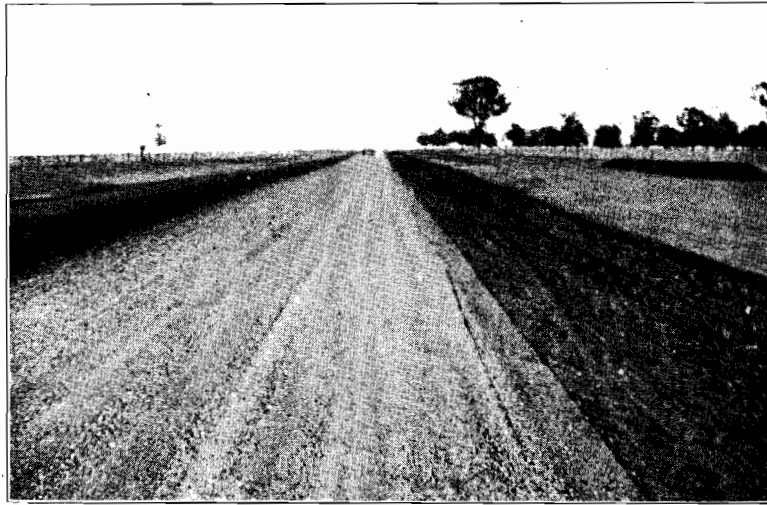
Plate No. 50.—Dunmunkle Shire, Marnoo-Rupanyup Road. Loam base with thin wearing course of crushed gravel.
