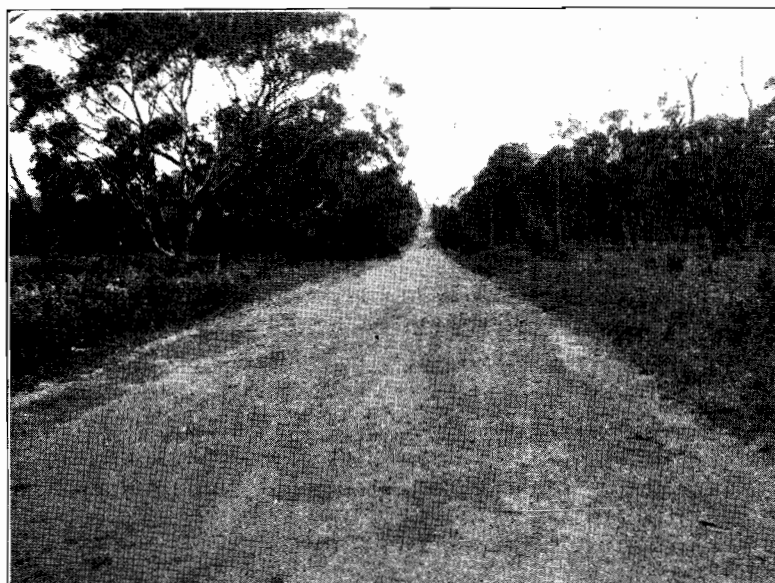
Plates Nos. 3 and 4.—Showing section of the Mornington to Flinders Road in 1913, and the same Section as it is to-day.
