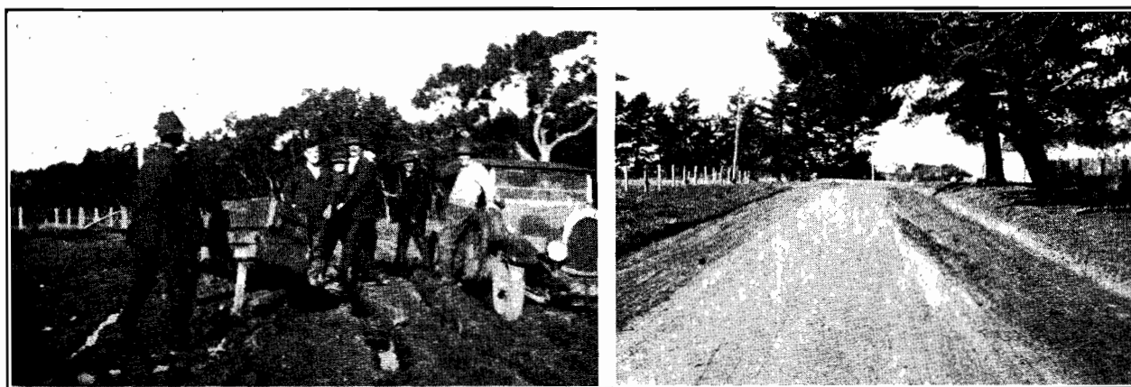
Plates Nos. 27 and 28.—Corinella Road.—(A) Road before construction. (B) Completed road.
