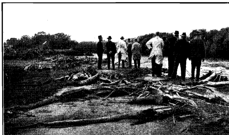
Plate No. 41.—Showing damage by floods on the Marlo Road.
