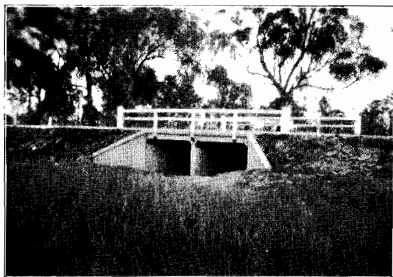
Plate No. 18.—Showing new culvert erected on the Hume Highway between Winton and Glenrowan.
