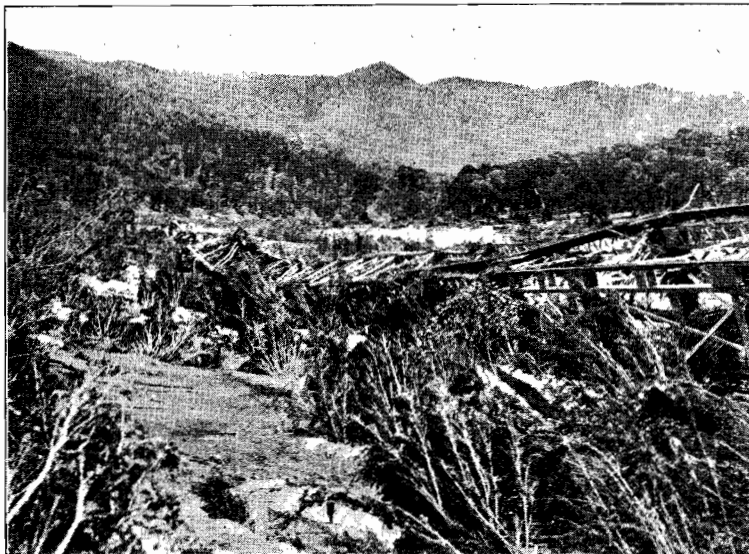
Plate No. 40.—Showing the effect of the flood and parts of the destroyed bridge at the junction of the Snowy and Deddick Rivers.
