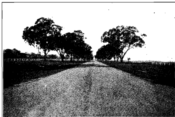
Plate No. 3.—Showing section of the Murray Valley Highway maintained with power-grader.
