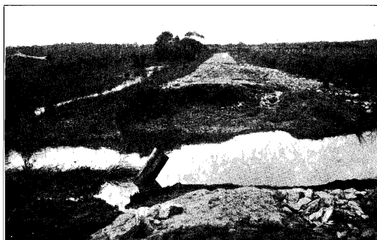
Plate No. 14A.—Showing damage on McCraw's Road, Korumburra Shire.
