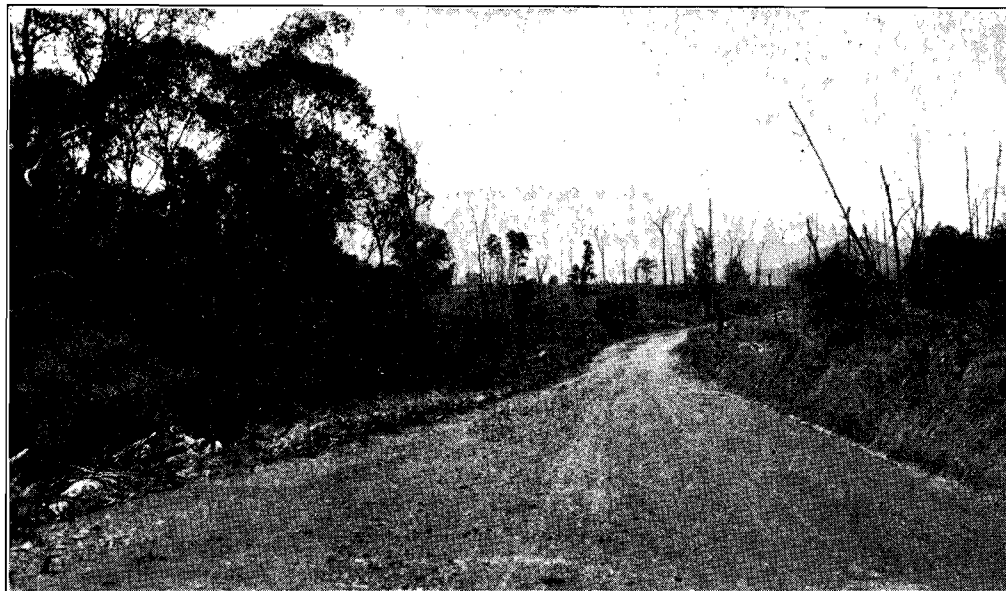
Plate No. 8.—Rose River Road near Dondangadale.
