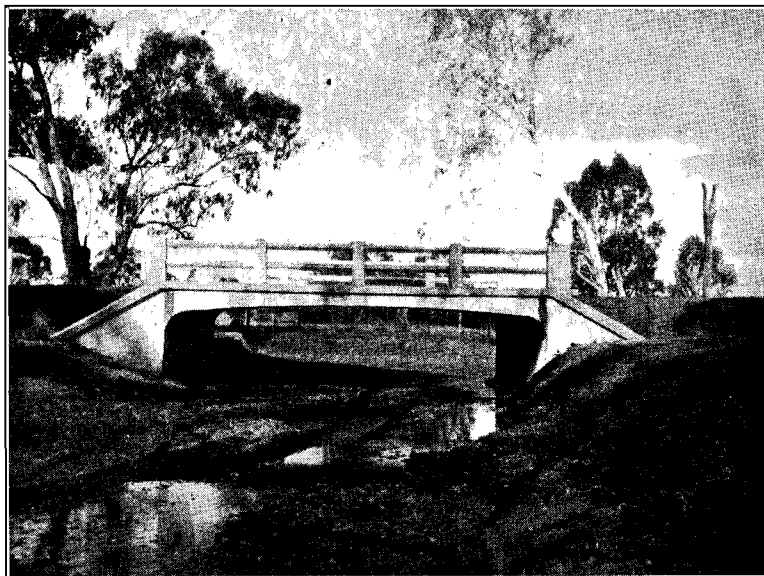
Plate No. 18.—Showing new bridge erected on the Calder Highway, north of Wedderburn.
