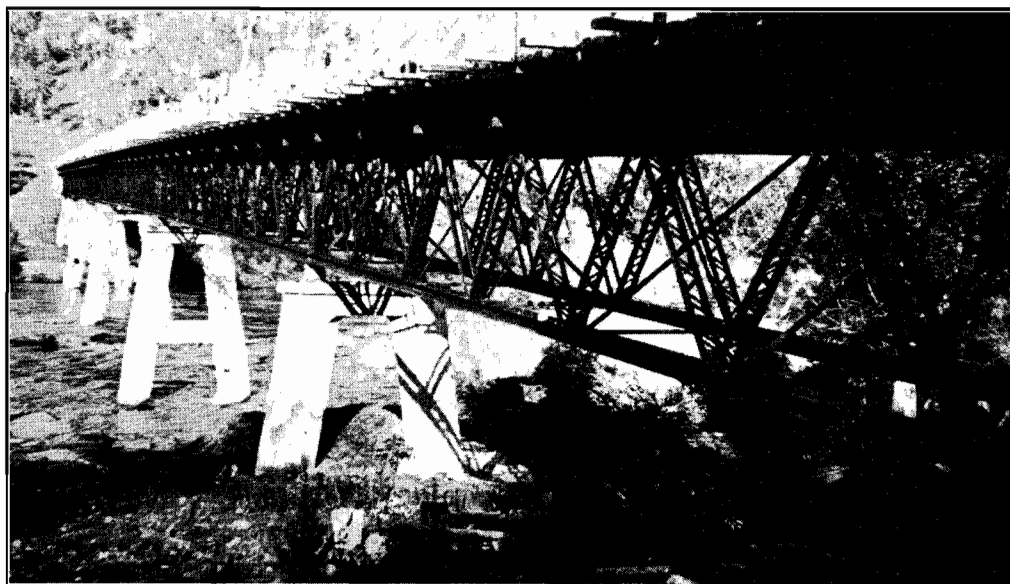
McKillop Bridge—Previous Structure.
