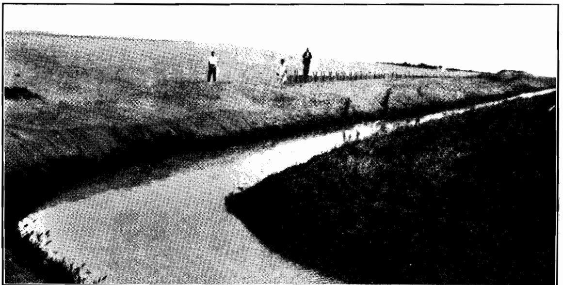
Water Channel, Piangil.—Sand drift from fallow shown encroaching on a running channel. No drift has occurred on opposite side where land is covered with vegetation.
