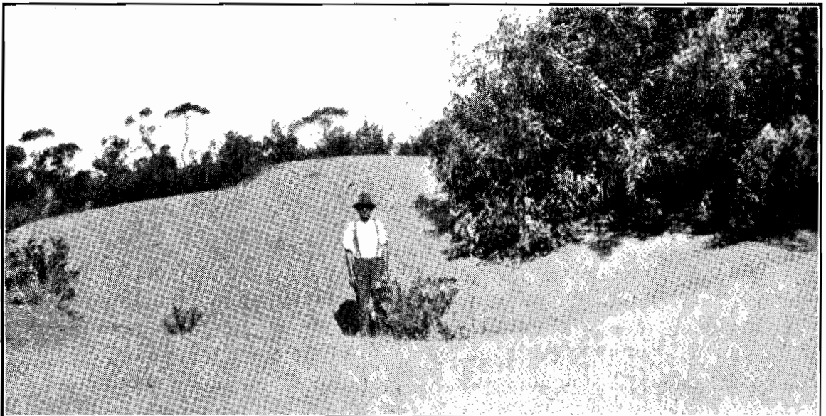
Tyrrell West Main Water Channel, near Sea Lake, completely blocked. 7,000 persons depend on this channel for their water supply.
