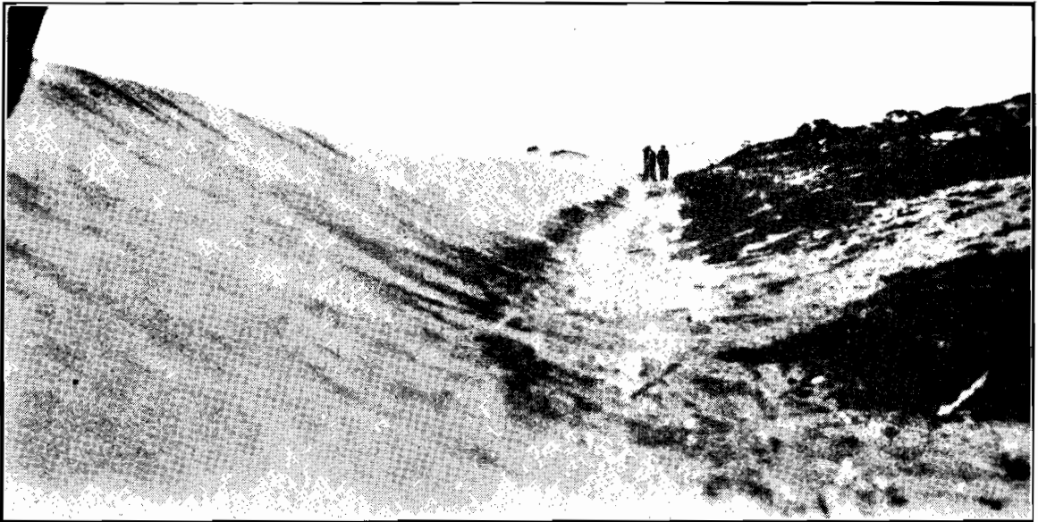
Water Channel, Tyrrell West.—Drift caught by channel banks. Channel which was originally 3 ft. bed width and 1 ft. 6 in. deep has had to be abandoned.
