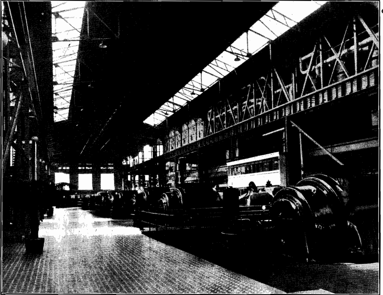
Yallourn Power Station, Turbine Room. The installed capacity (125,000 kw. in six 12,500 kw. sets and two 25,000 kw. sets) is to be increased progressively to 200,000 kw., by the provision of two further 25,000 kw. sets and two 12,500 kw. sets, the latter to be high pressure.
