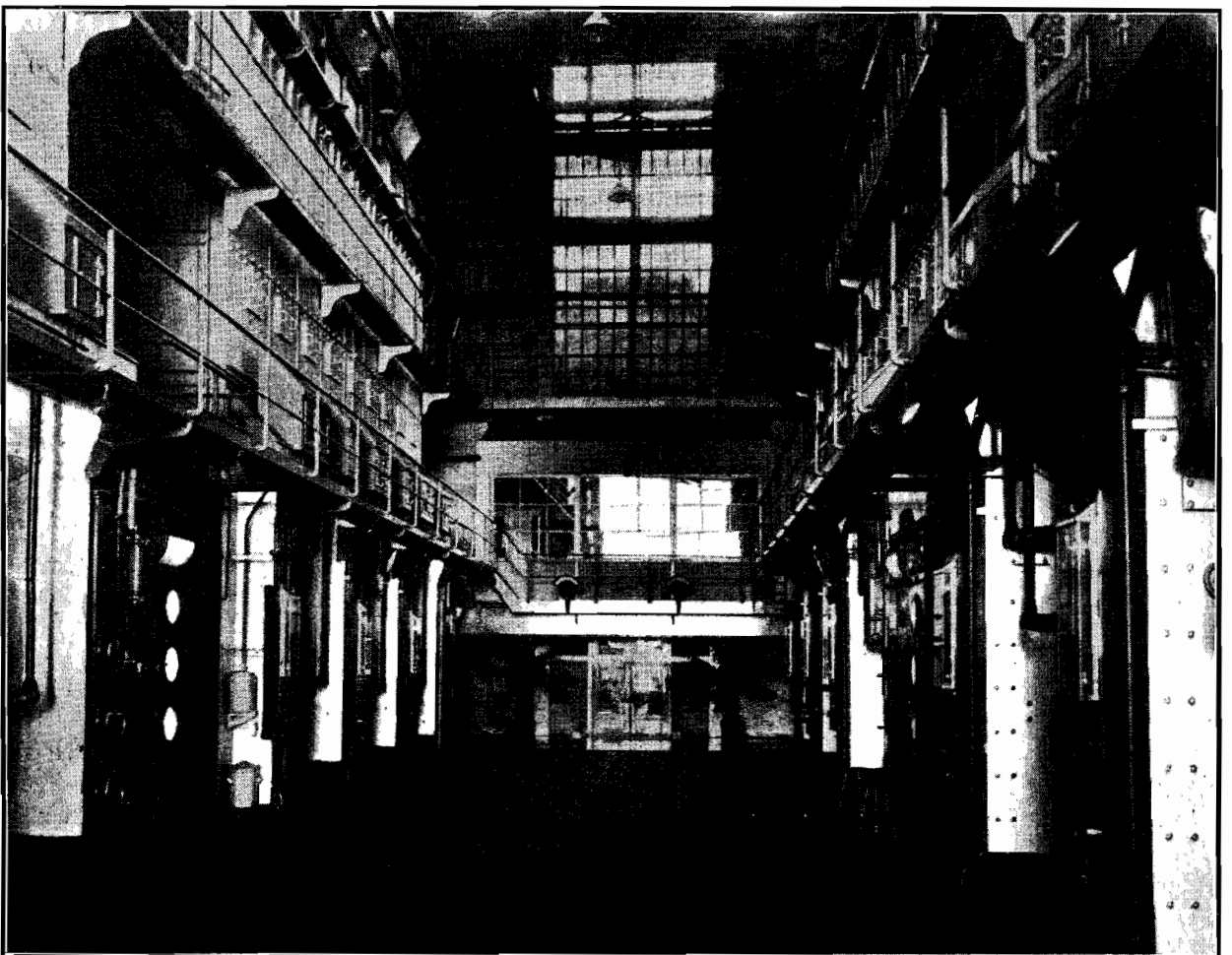
• Yallourn Power Station, No. 2 Boiler House, showing four (pressure and temperature 250 lb. and 650° F. respectively) of the ten boilers to be installed to complete the installation. The remaining six boilers will operate at a pressure and temperature of 650 lb. and 900° F. respectively.
