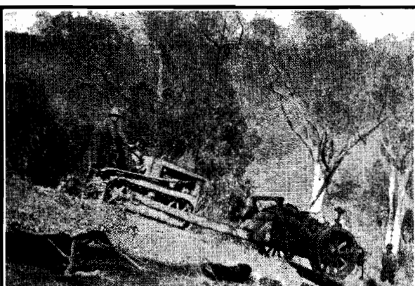
Caterpillar Tractor descending same grade after being attached to wire rope, by which trailer was drawn up the hill as tractor descended.
