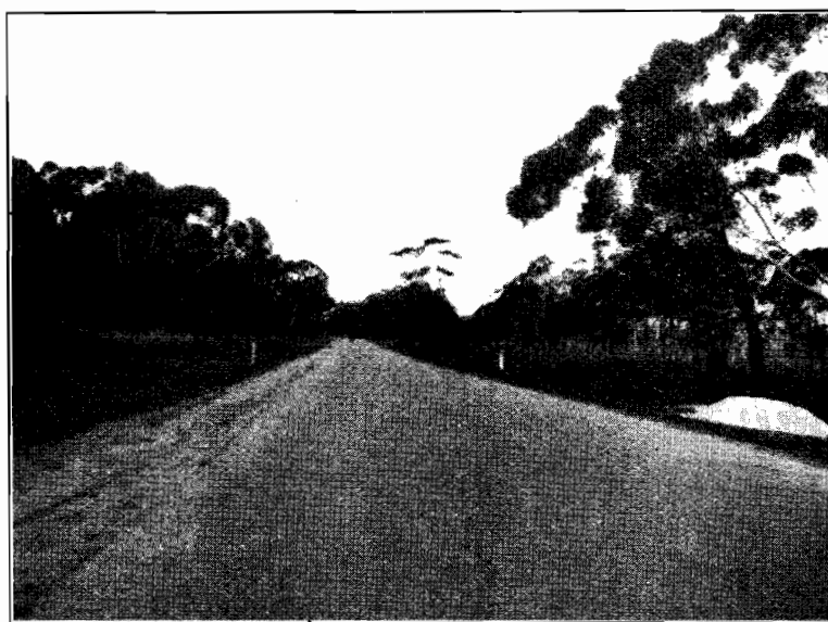
Plate No. 2.—Western Highway near Wallace, showing reconditioned surface
