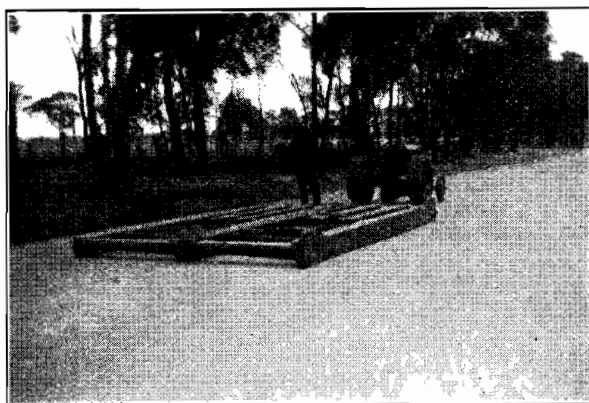
Plate No. 1.—Hume Highway. Surface treatment with road planers, between Longwood and Euroa.
