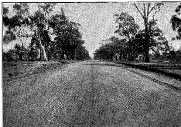
Plate No. 19.—Sprayed Road Pavement between Avenel and Longwood, consisting of granite or natural earth selected from borrow pits on the roadside during forming.
