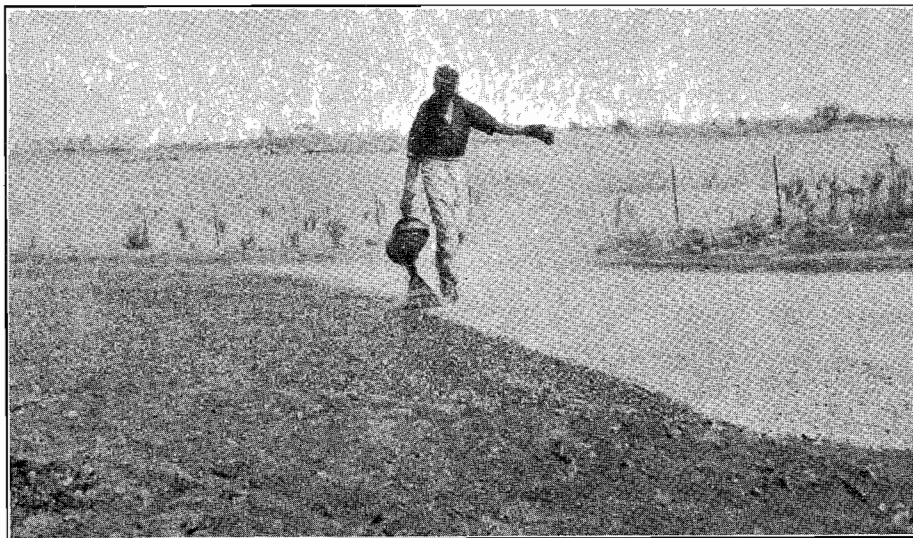
Plate No. 14.—Application of bitumen to consolidated stone in the construction of bituminous macadam surfacing. One gallon per square yard.
