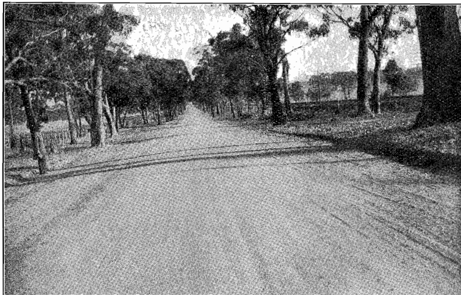
Plate No. 12.—Hume Highway. Gravelling carried out between Seymour and Avenel.
