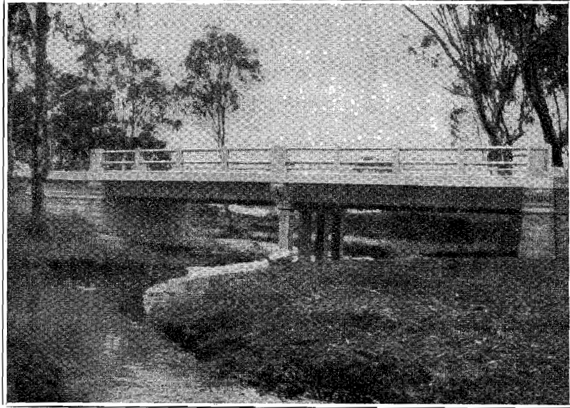
Plate No. 19.—Honeysuckle Creek bridge, near Baddaginnie, Hume Highway, Section 2. Showing old masonry abutments.
