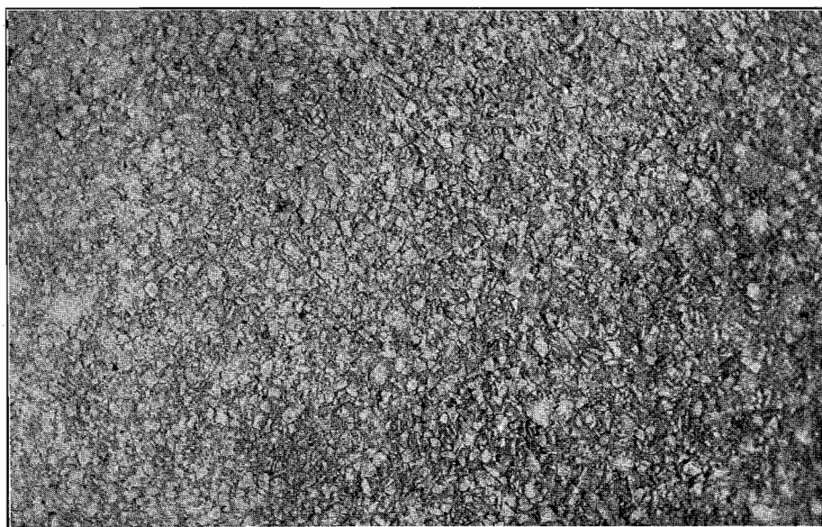
Plate No. 15.—Bituminous macadam surfacing immediately before sealing.
