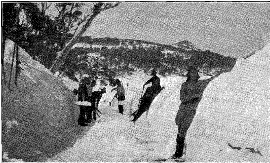
PLATE NO. 9.—Mount Buffalo-road under Winter Conditions. Removing Snow from Formation.
