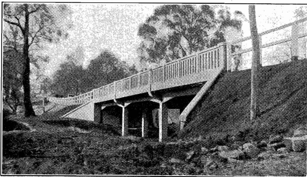
PLATE No. 8.—Portion of Bridge over Woori Yallock Creek.
