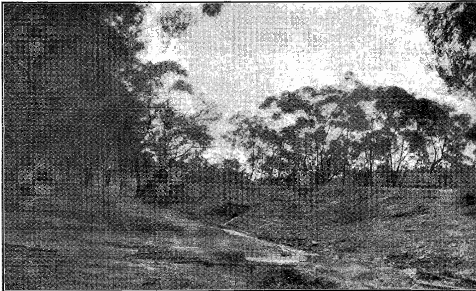
ILLUSTRATION No. 2.—Old formation and Granite Culvert near Avenel.
