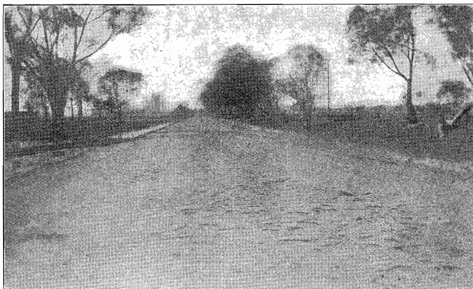
ILLUSTRATION NO. 5.—North-Eastern Highway near Benalla, showing cobble stones.
