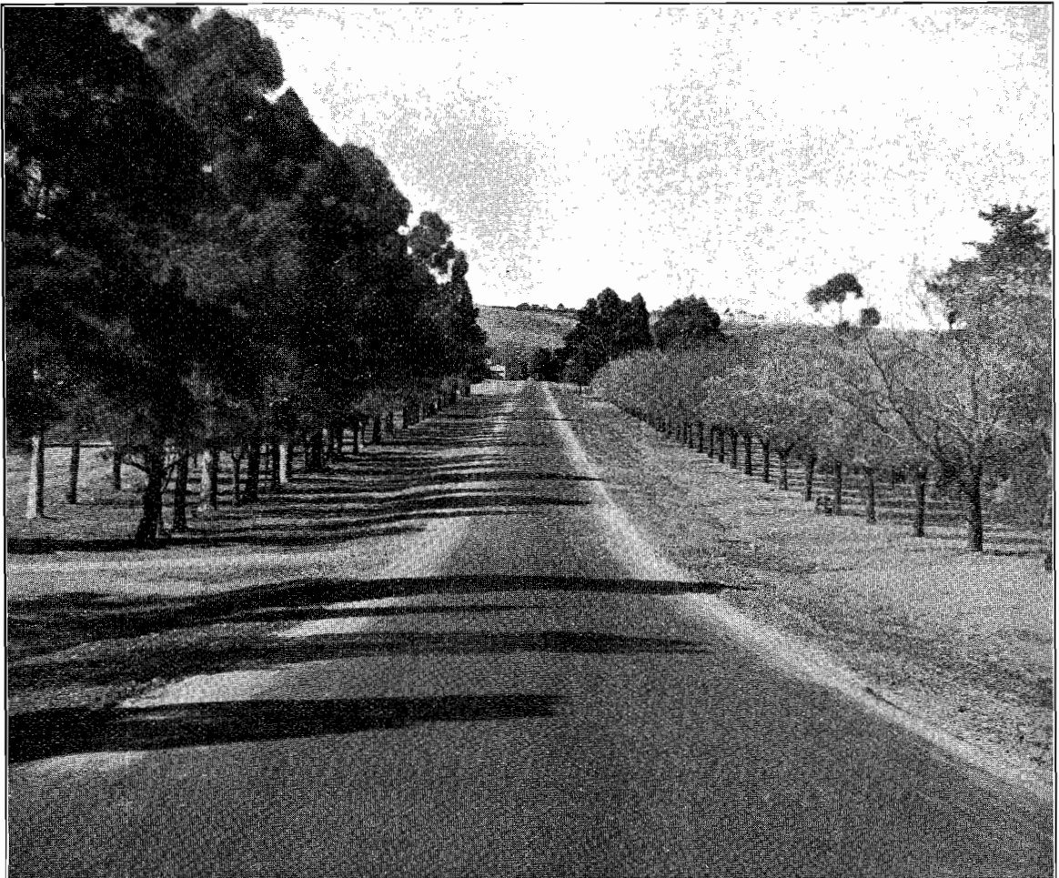
PLATE NO. 2.—Reconstructed section of North-Western Highway at Keilor.
