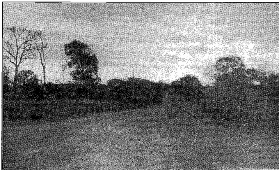
ILLUSTRATION No. 6.—Re-shaped gravel road near Winton—scarified sides.
