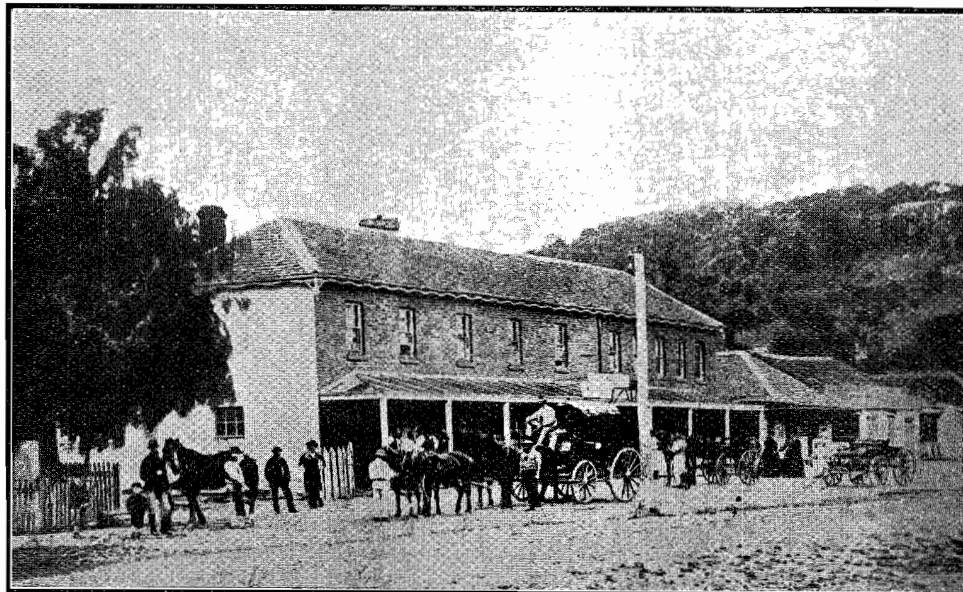
ILLUSTRATION No. 3.—Former Settlement at Longwood.
