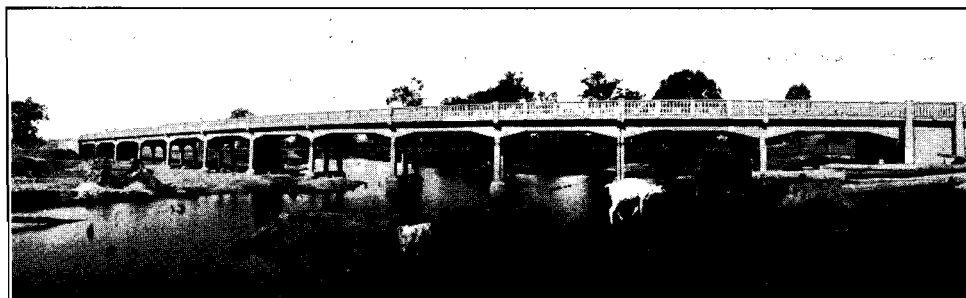
Bridge at Wodonga in Murray basin—Main Sydney Road.
