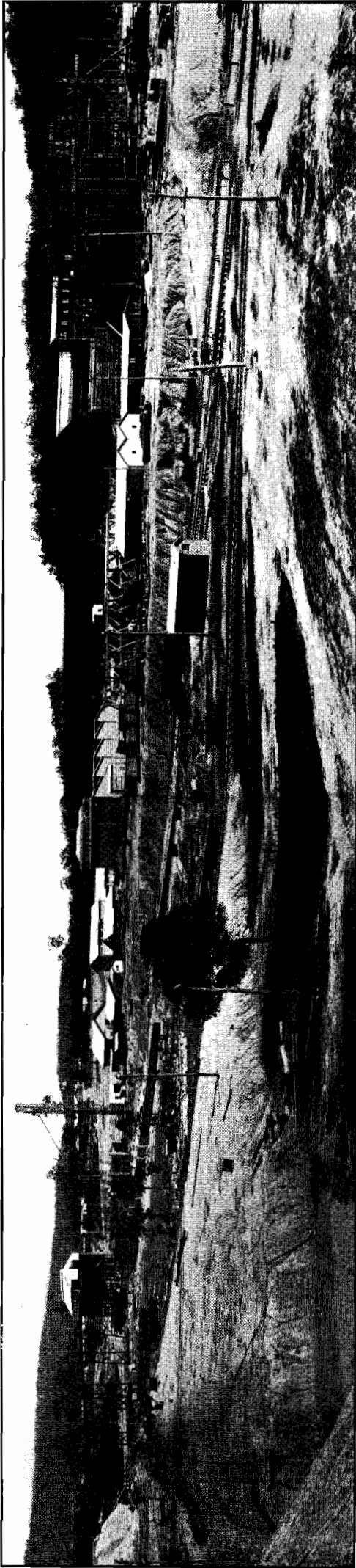
1. The Power Station Area, Yallourn.—On the right are the power station buildings showing portion of the turbine house in an advanced stage of completion, with the structural steel work of the boiler house in course of erection. The Main Workshops, Stores, &c., appear in the centre, and on the left is the coal crushing and screening house.
