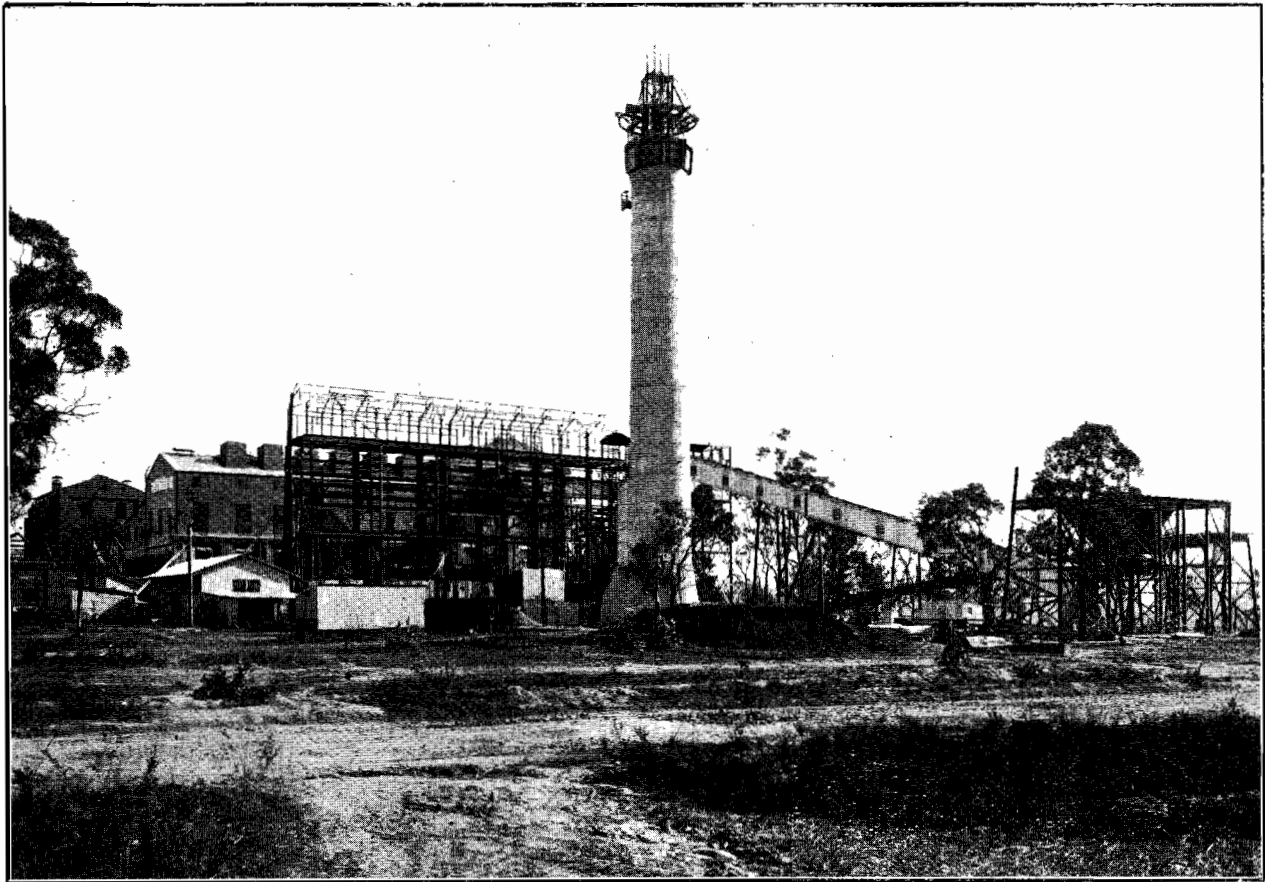
3. Briquetting Factory, Yallourn, showing structural steel for turbine and boiler house in course of erection. The concrete chimney will be 320 feet in height when completed.
