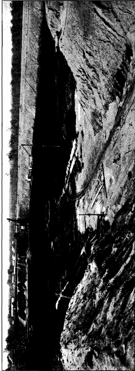
2. The Open Cut, Yallourn.—In the centre is one of the large Bucyrus shovels engaged in the process of overburden removal. The coal vertically under the area from which the overburden has been stripped is estimated at 2,000,000 tons.
