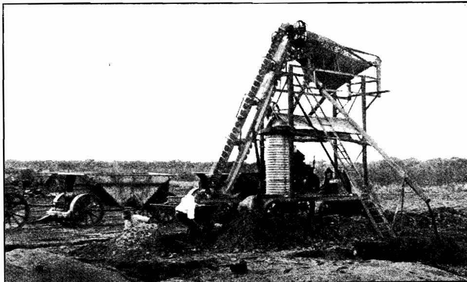
Plate 9. Screening Plant, Shire of Mildura.
