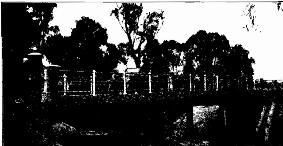
Plate 8. Yarrawonga Road, Rutherglen Shire.
