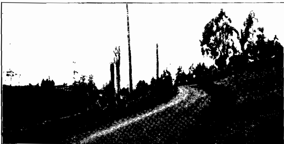
Plate 4. Ferntree Gully-Olinda Road (completed).
