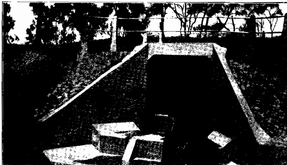
Plate 7. Culvert, Castlemaine-Bendigo Road.
