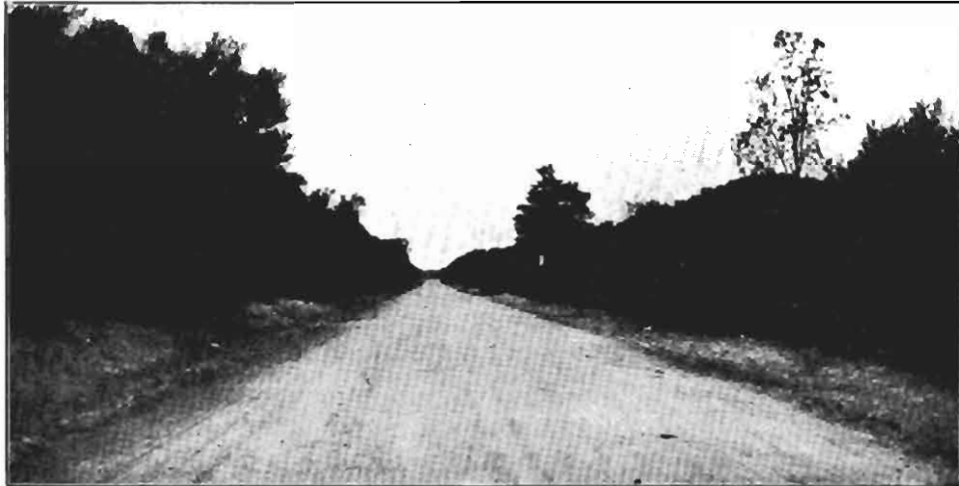
Plate 20. Showing excellent road surface of Macadam obtained by efficient rolling with steam roller, Shire of Frankston and Hastings.
