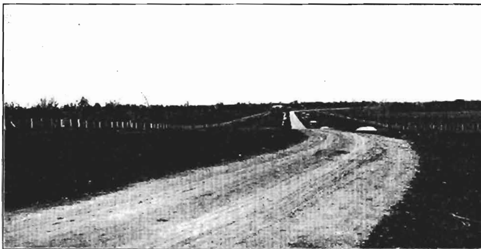
Plate 22. Completed section Hopetoun-Woomelang Road, Shire of Karkaroc.
