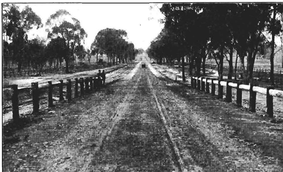
Plate 15. Restored section Sydney Road, between Benalla and Wangaratta—Shire of Benalla.
