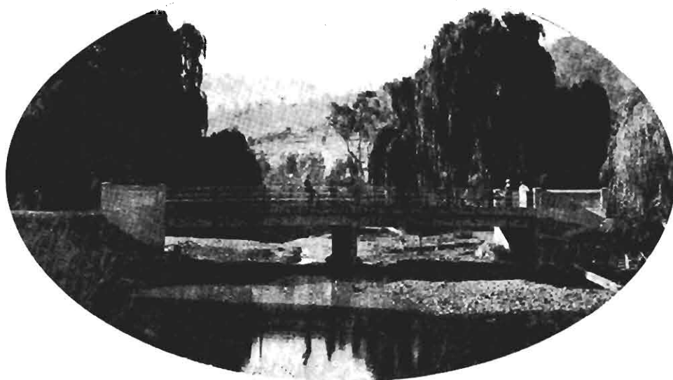
Plate 16. New reinforced concrete bridge at Bright.
