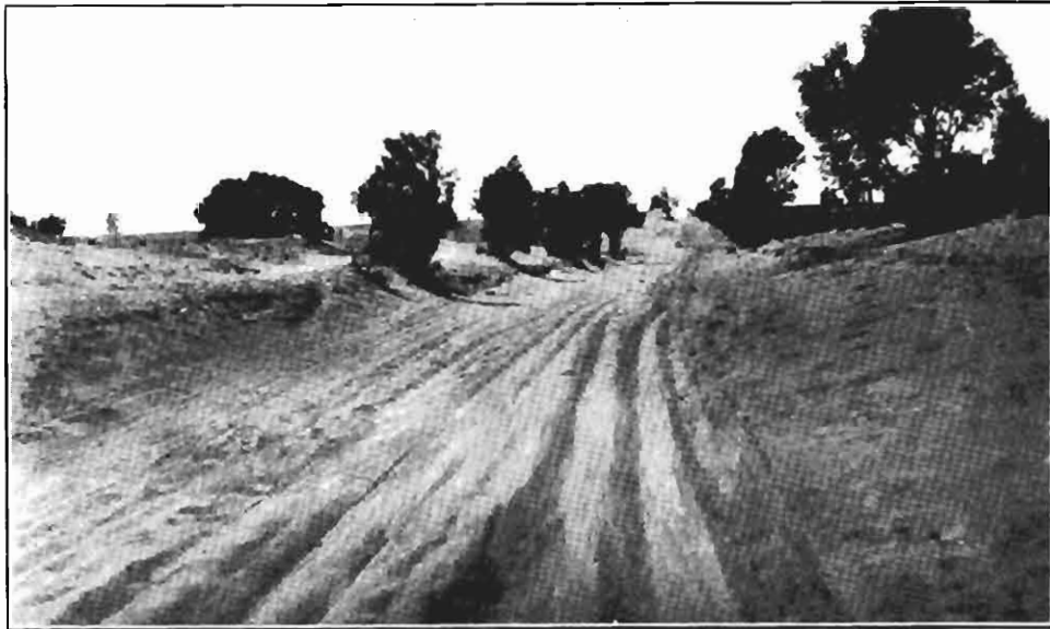
Plate 2. Showing sand drifts in cutting.
