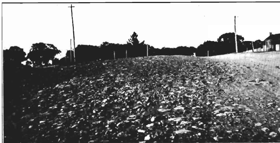
Plate 7. Showing neglected section, Melbourne-Bendigo Road, now being re-constructed.
