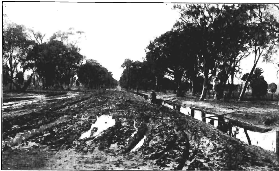
Plate 14. Section of Sydney Road known as "Gluepot," now being restored—Shire of Benalla.
