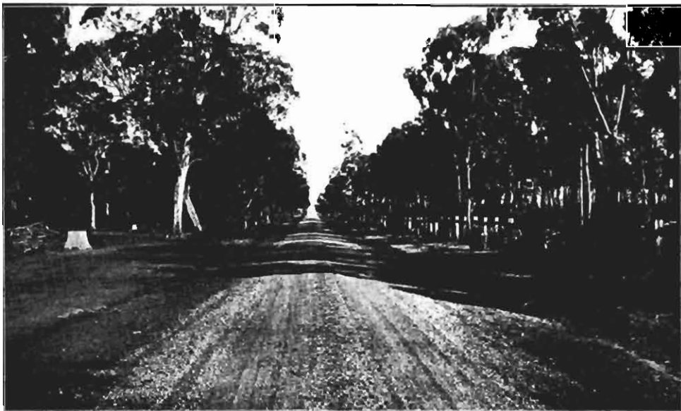
Plate 13. Completed gravelled section, Main Gippsland Road at Providence Ponds, Bairnsdale Shire.
