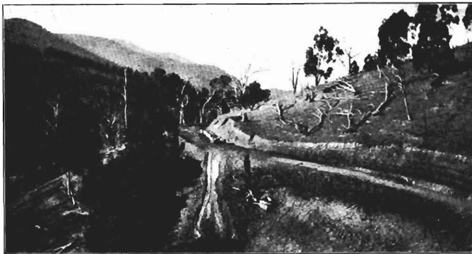
Plate 27. Showing graded deviation in progress, Omeo Shire.
