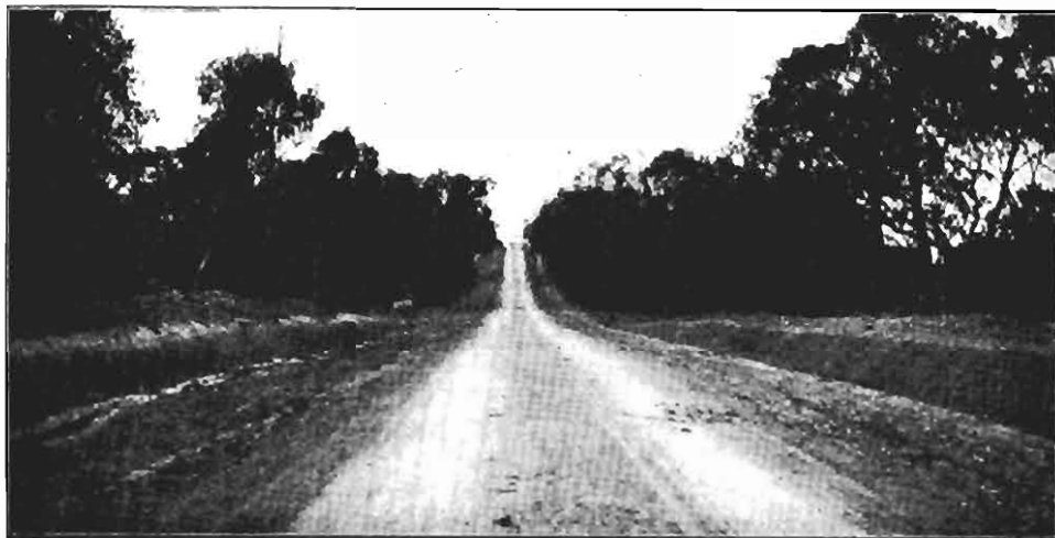
Plate 21. Completed section Frankston-Flinders Road, Shire of Frankston and Hastings.
