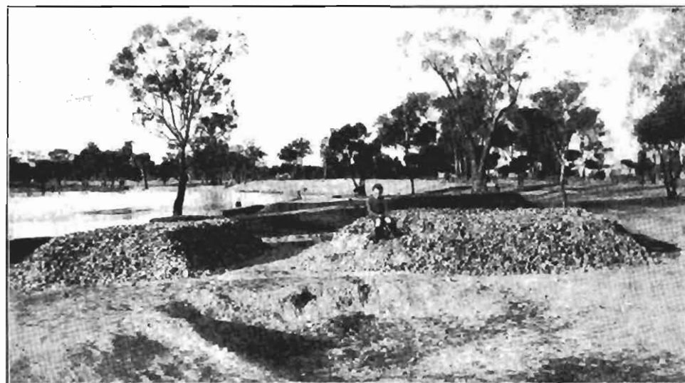
Plates 24 and 25. Showing heaps of ironstone taken from bed of Murray River at Mildura for Mildura-Wentworth Road.
