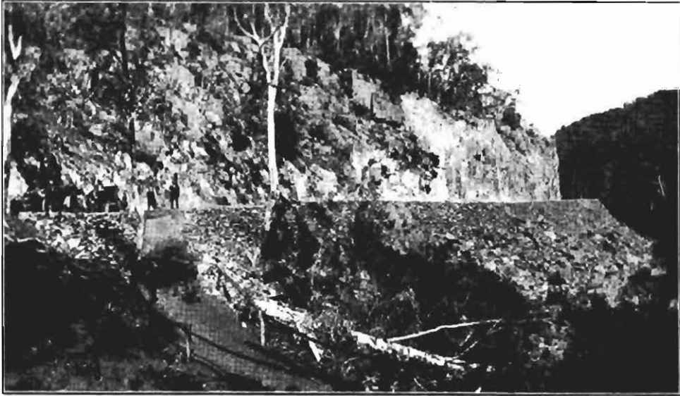
Plate 12. Showing easy gradient obtained by side cutting, Dargo Road.
