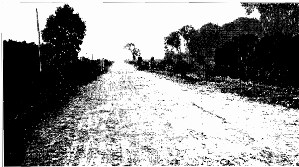
Plate 53. Shire of Phillip Island and Woolamai. Showing road constructed of burnt clay; in use over 35 years.
