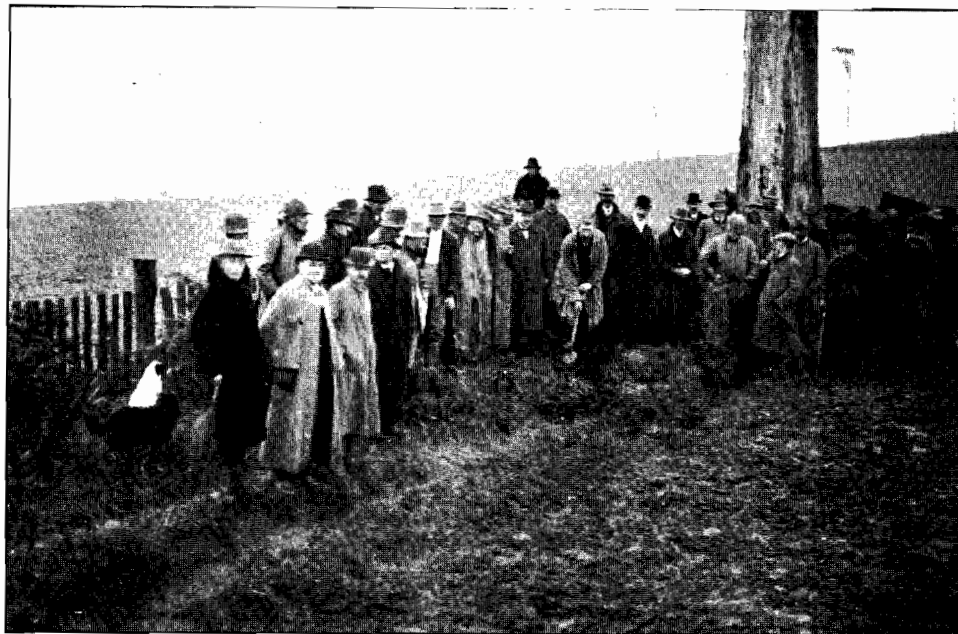
Plate 76. Commencing a new work. The Honorable F. Hagelthorn, Minister of Public Works, turning the first sod, Bear Creek Deviation, Shire of Warragul.
