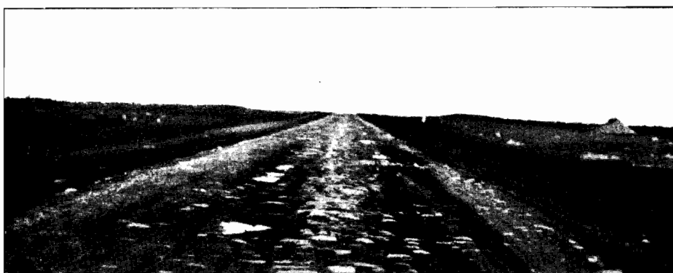
Plates 28 and 29. Showing sections of Melbourne-Geelong road, with foundations exposed through neglect of maintenance.
