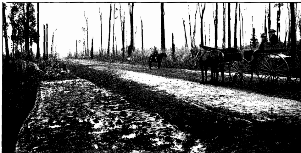
Plates 78, 79, and 80. Showing road works in Gippsland--Woorayl Shire. (1) Early stages of the work. (2) Contractor's portable stone-breaking plant. (3) Finished roadway.
