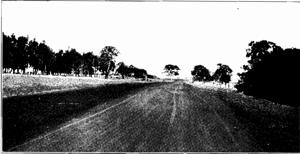
Plate 44. Mortlake Shire, showing fine stretch of Mortlake-Lake Bolac road, near Woorndoo, constructed of ironstone gravel.
