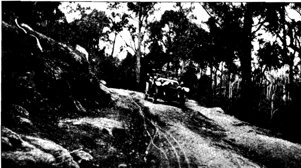
Plate 22. Section of road over Mount Taylor, between Bairnsdale and Bulumwaal.
