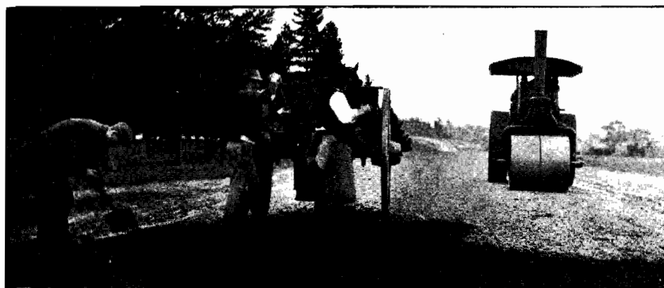
Plates 54 and 55. Showing earthy material and weeds being taken from water tables and spread on metalled roads.
