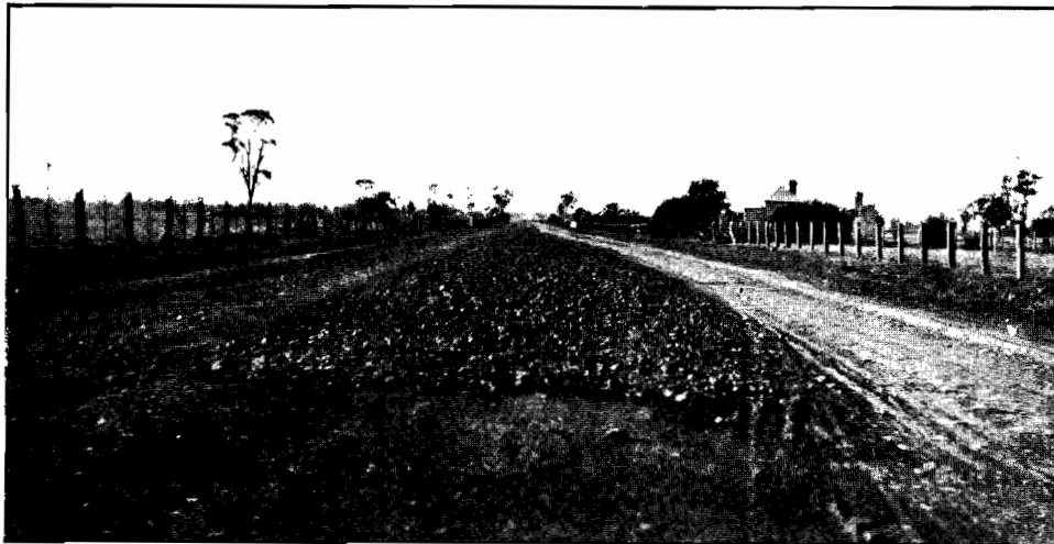
Plates 64, 65, and 66. Showing material spread or dumped on roads without rolling.
