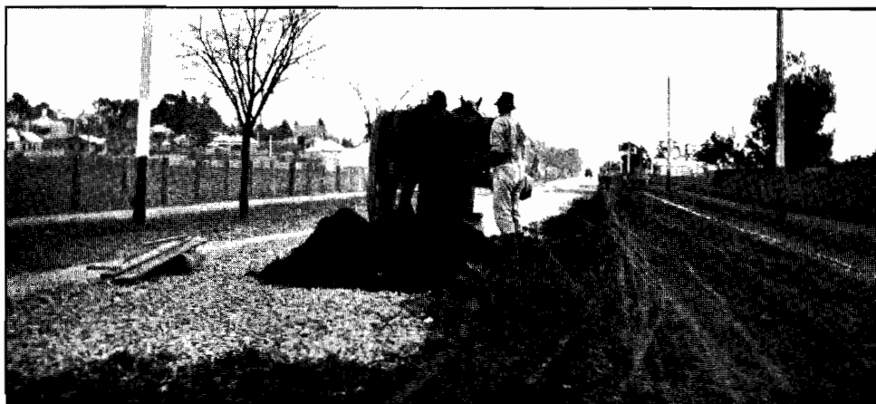
Plates 56 and 57. Showing earthy material and weeds being taken from water tables and spread on metalled roads.
