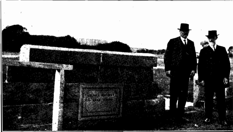
Plate 39. Showing remains of old stone culvert constructed by Belfast District Roads Board, 1856.
