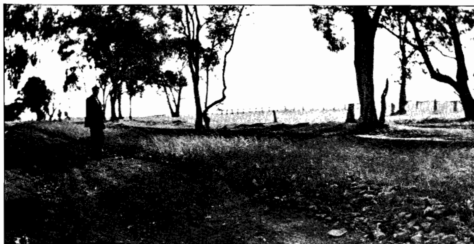
Plate 35A. Section of main Sydney-road, illustrating wasteful and useless method of construction. Note crop of grass and size of metal. To avoid this the traffic uses the near side of road to left of figure.
