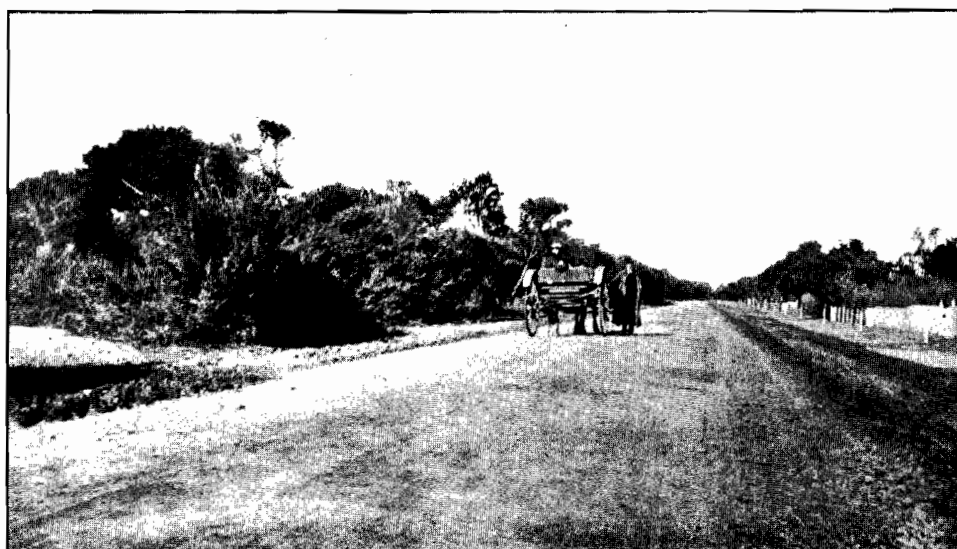
Plate 81. Showing completed section of Point Nepean-road between Mordiallee and Frankston.
