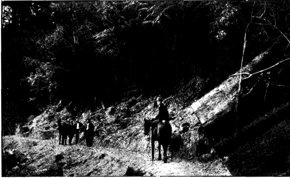
Plate 33. Showing sharp bend and narrow side cutting on Beech Forest-Apollo Bay road.
