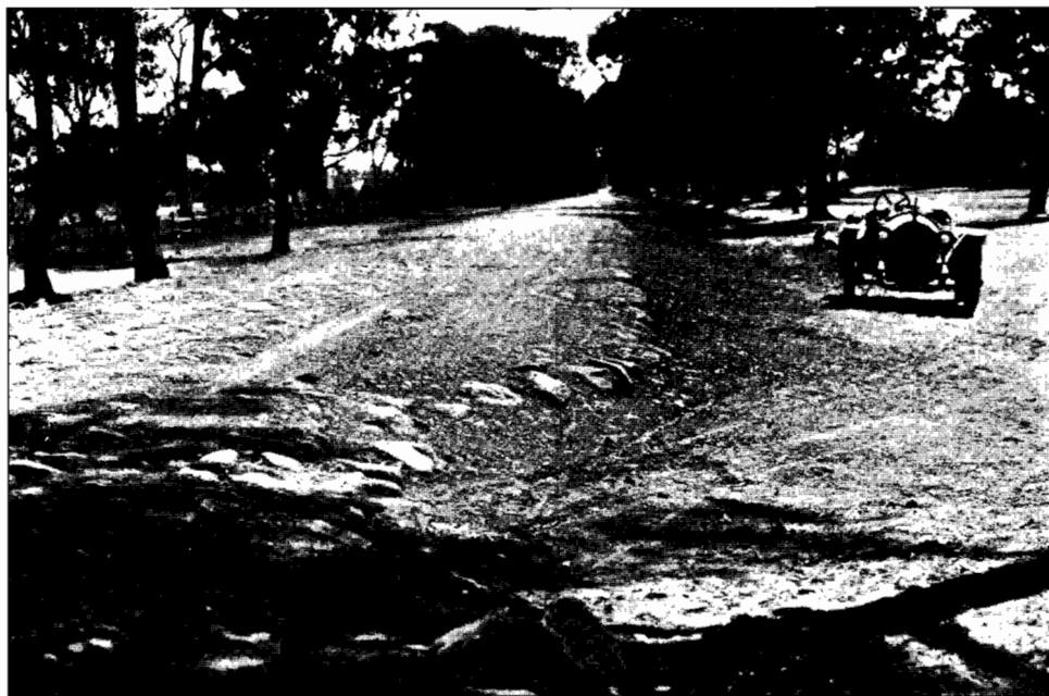
Plate 34. Section of Sydney-road, showing foundation stones exposed through neglect of maintenance.
