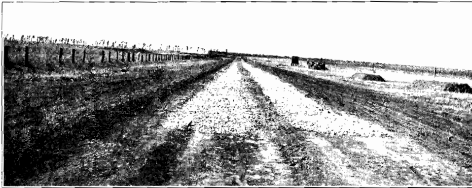
Plate 70. Showing road being repaired by the intermittent or annual system.
