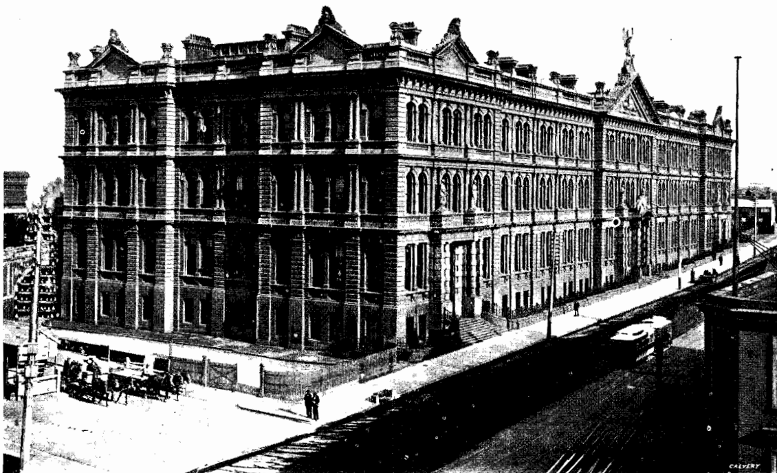
VICTORIAN RAILWAYS. RAILWAY OFFICES, SPENCER-STREET, MELBOURNE.
