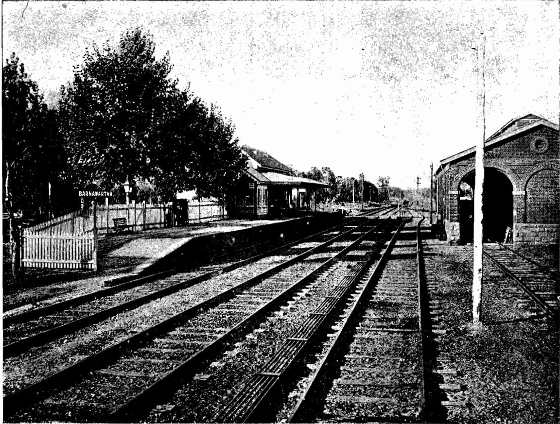
VICTORIAN RAILWAYS. BARNAWARTHA STATION.
