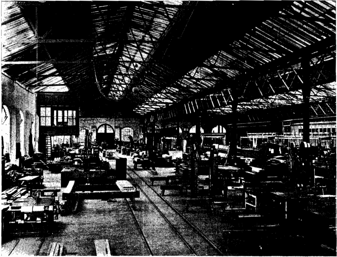
VICTORIAN RAILWAYS. CAR SHOP, NEWPORT.
