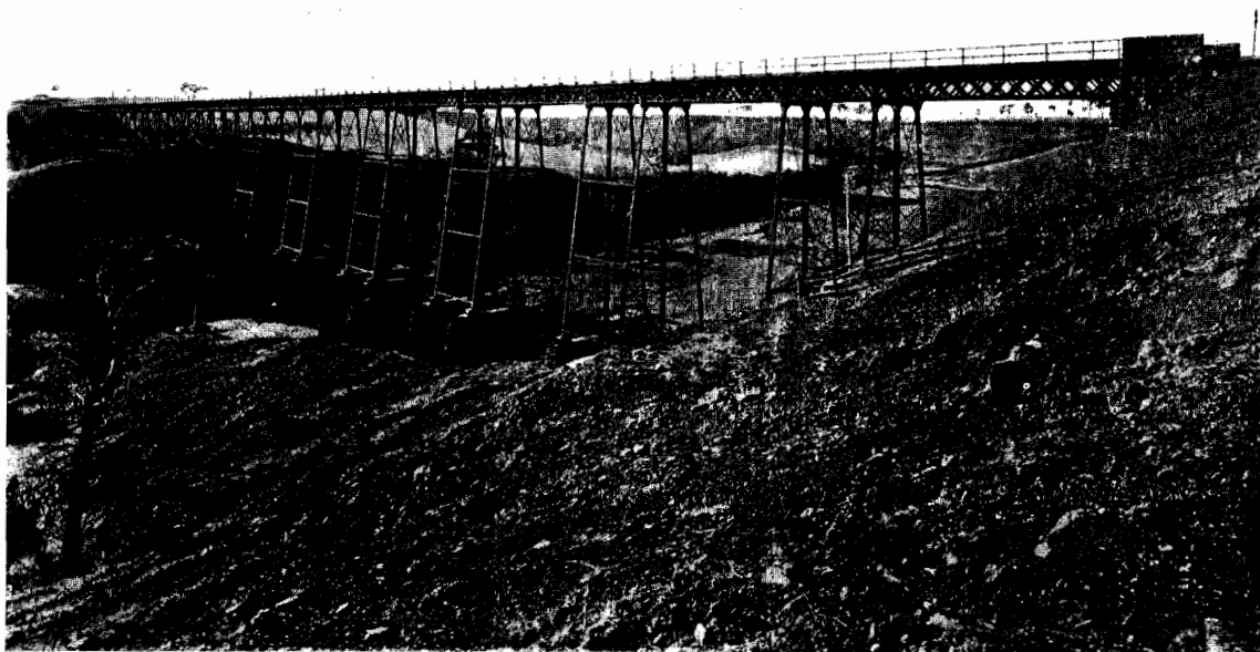
VICTORIAN RAILWAYS. WERRIBEE VIADUCT.
