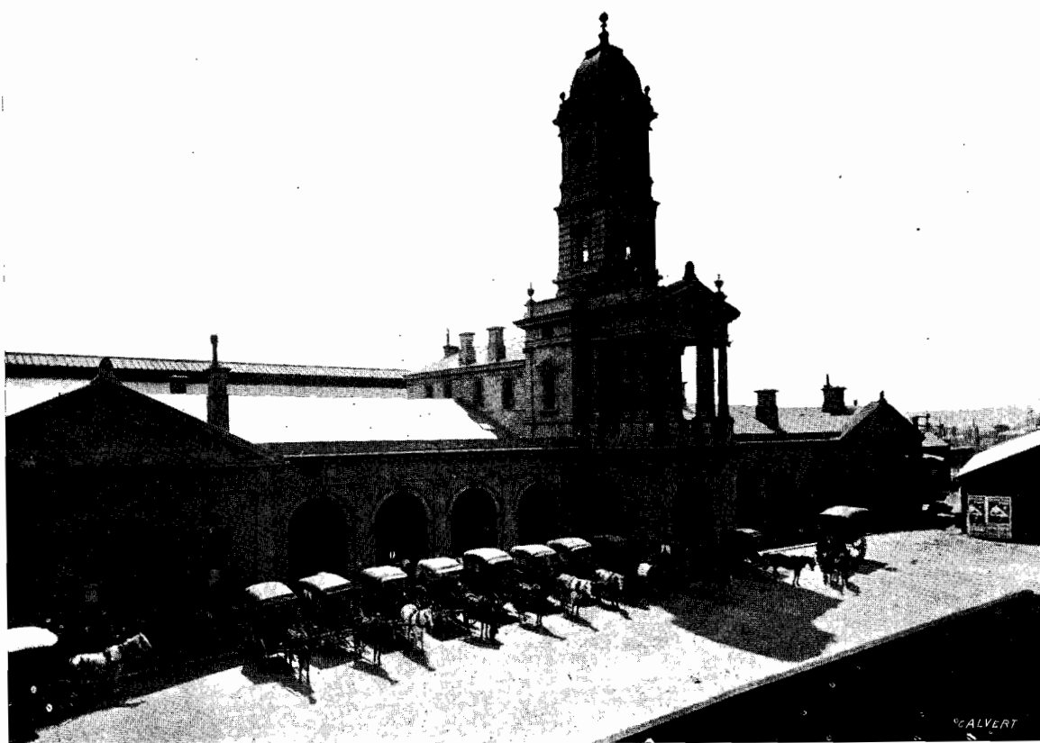
VICTORIAN RAILWAYS. BALLARAT STATION.
